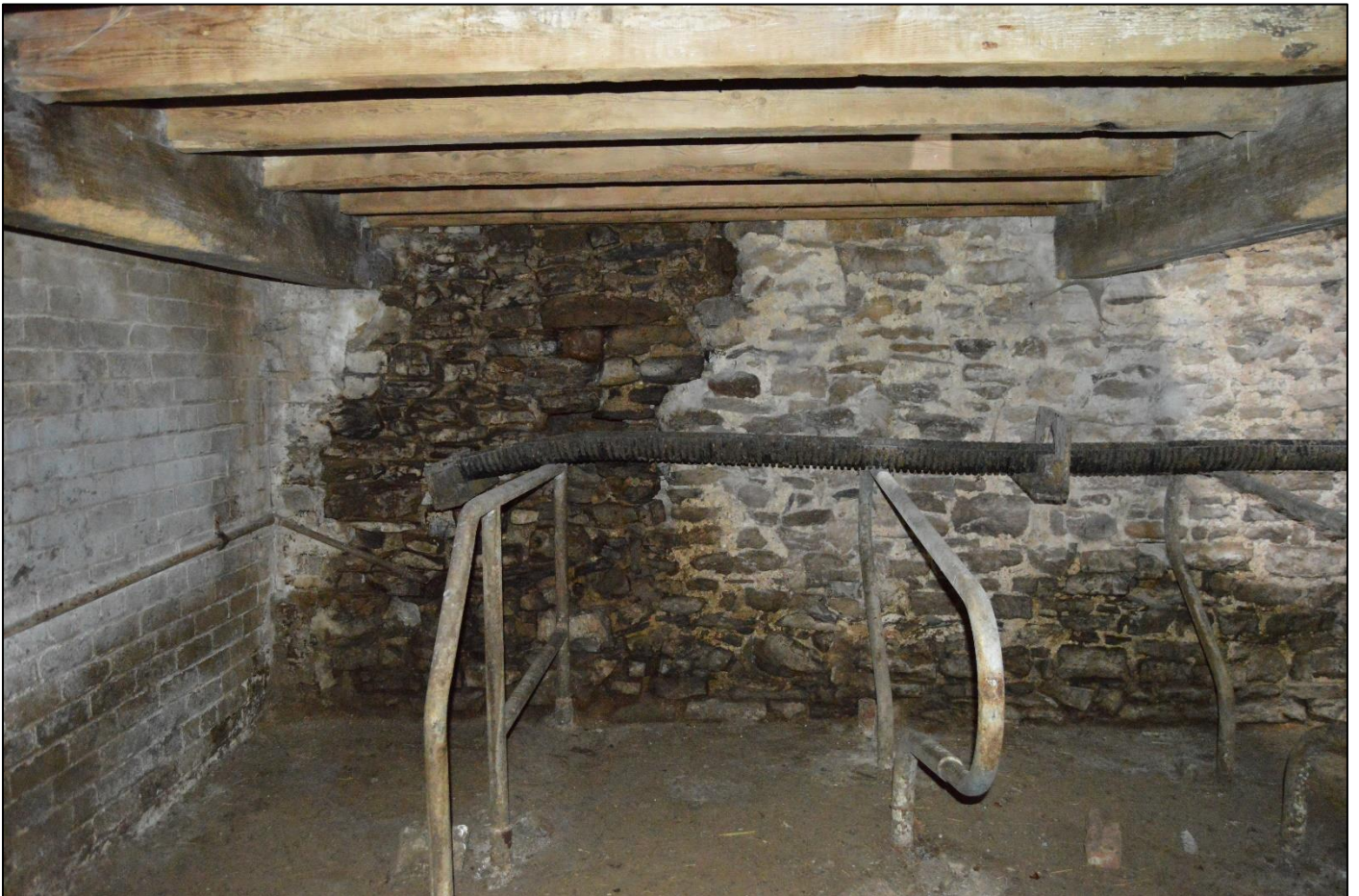
PL49: View north from below the west hay loft.
