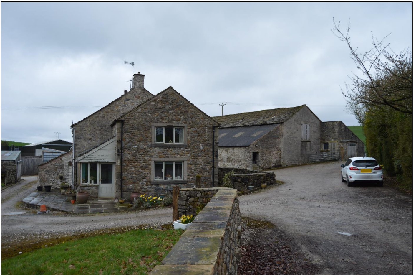
PL16: View towards the farmhouse and barn from the west.
