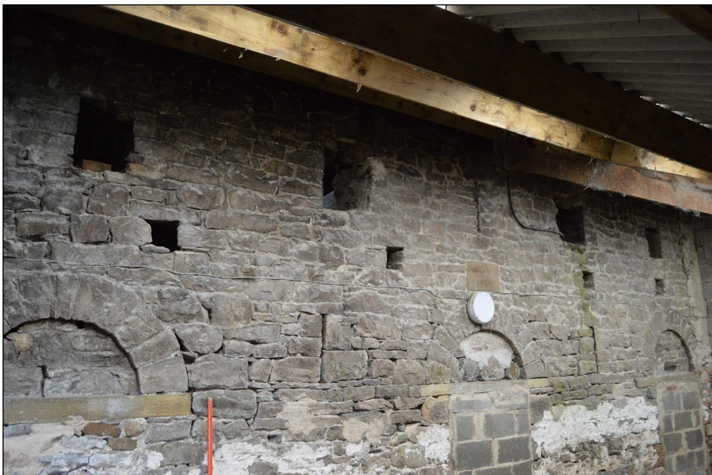
PL34: View of the 'breathers' to the north elevation of the original barn.
