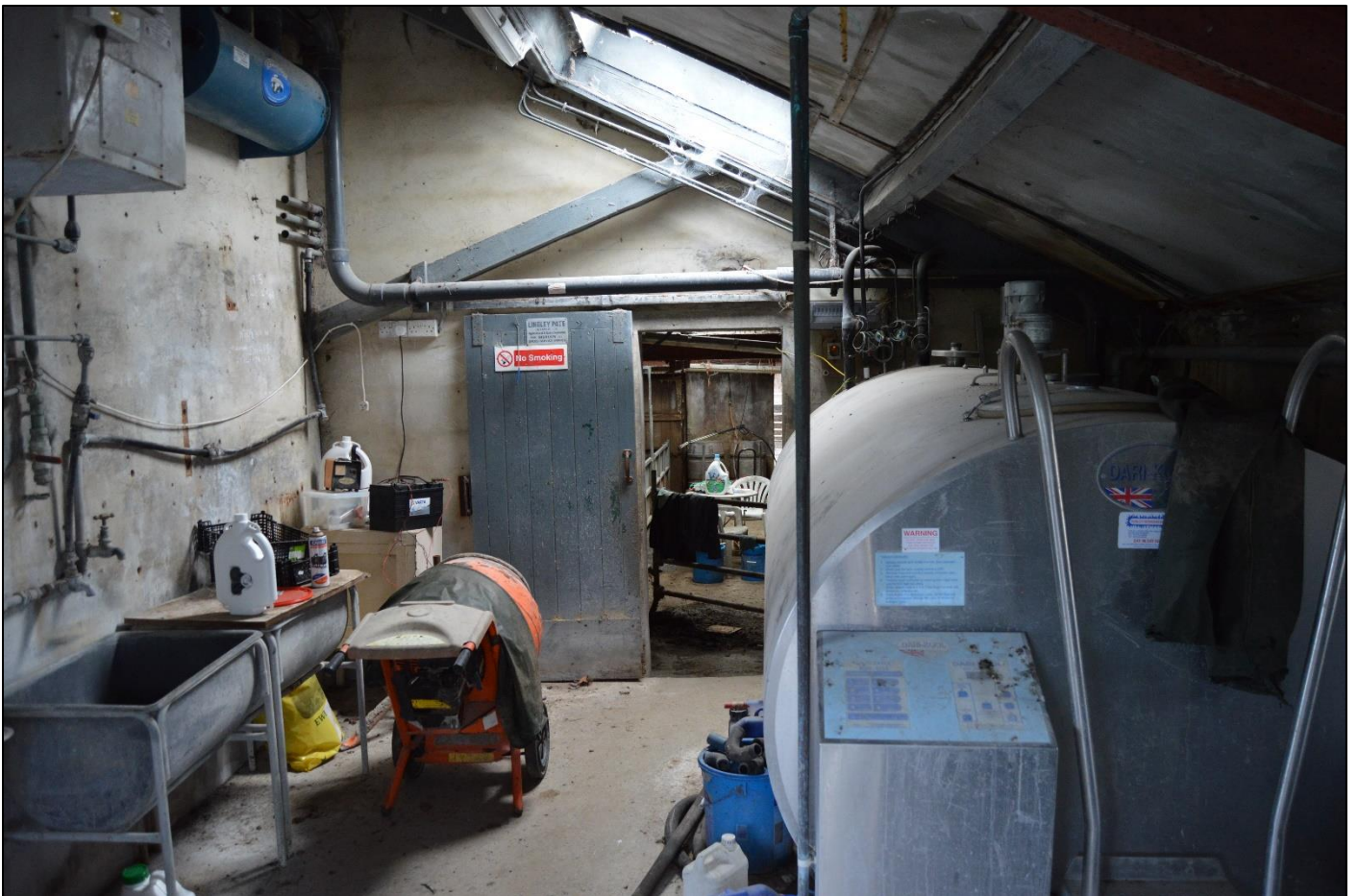
PL20: View east from within the west addition of the south outshut.
