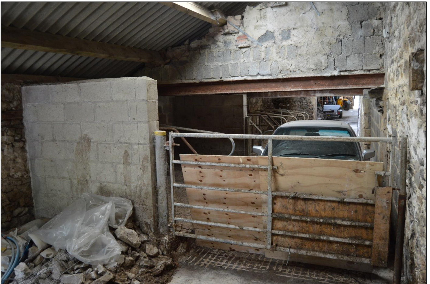
PL18: View east from the west end of the north outshut.
