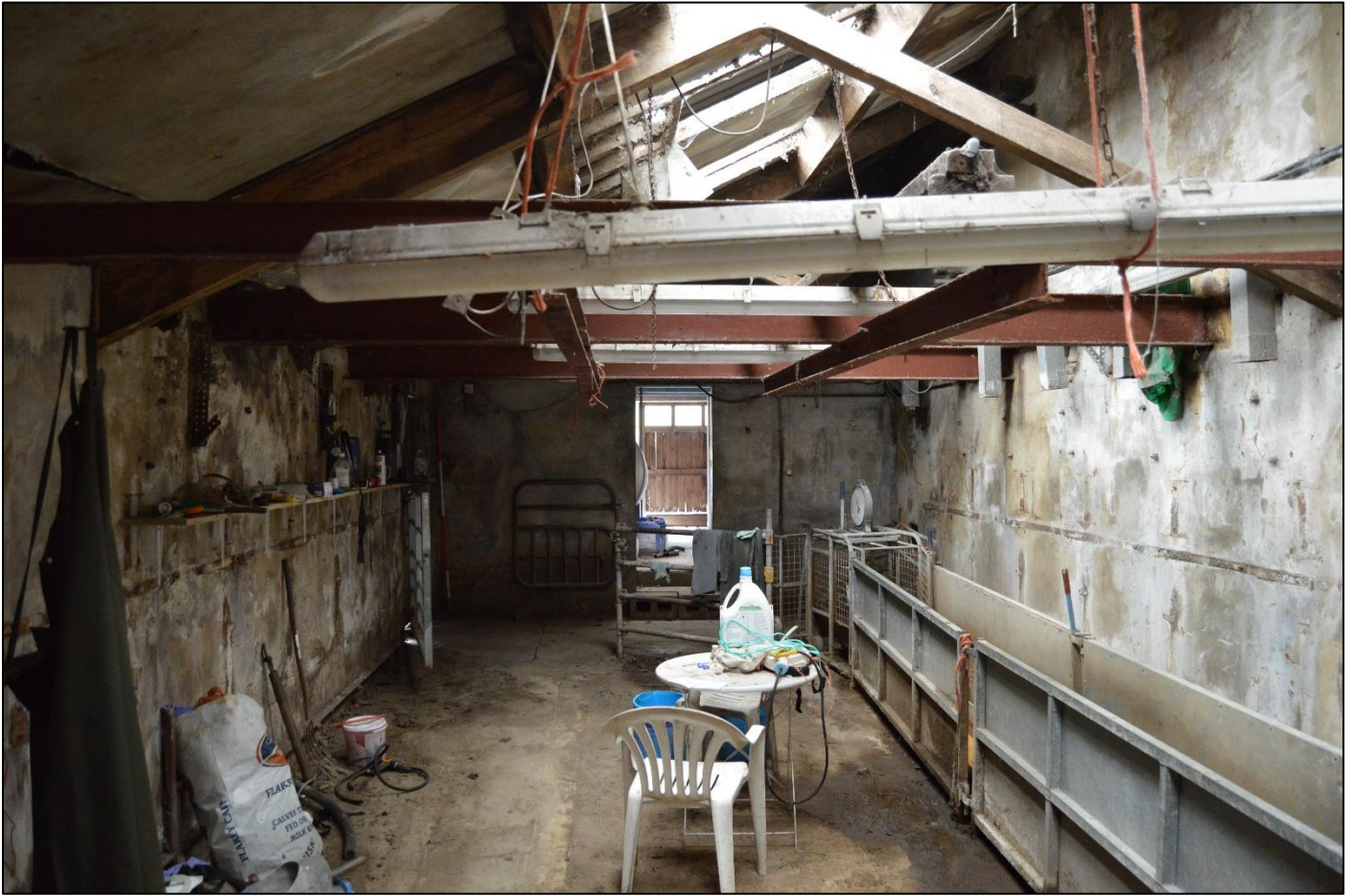
PL21: View west within the south outshut.
