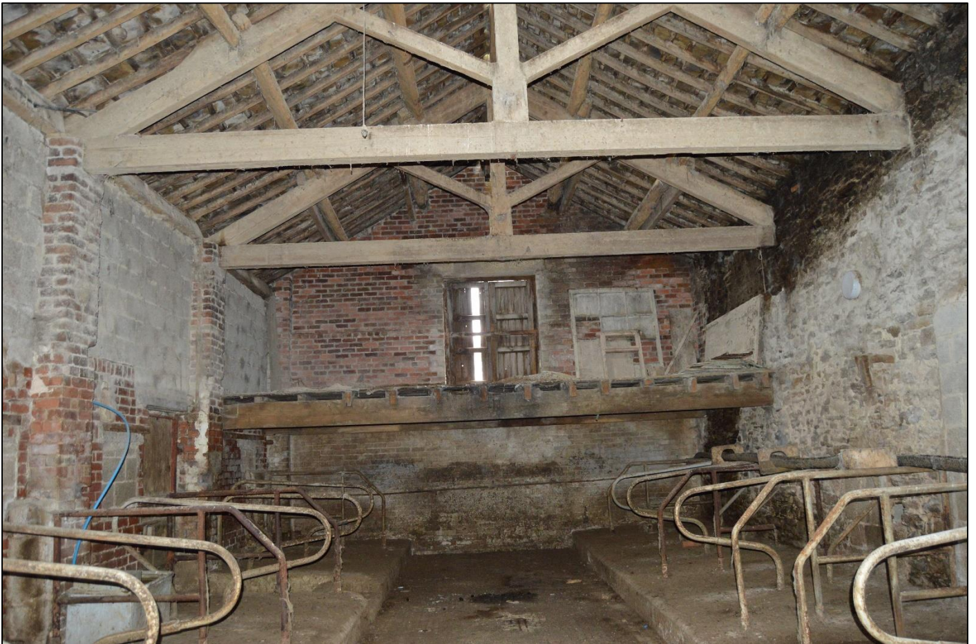
PL40: View west within the original barn.
