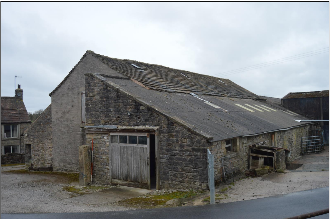
PL06: View of the barn from the south west.
