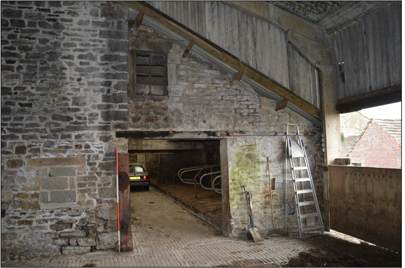
PL25: View of the east elevation of the north outshut.
