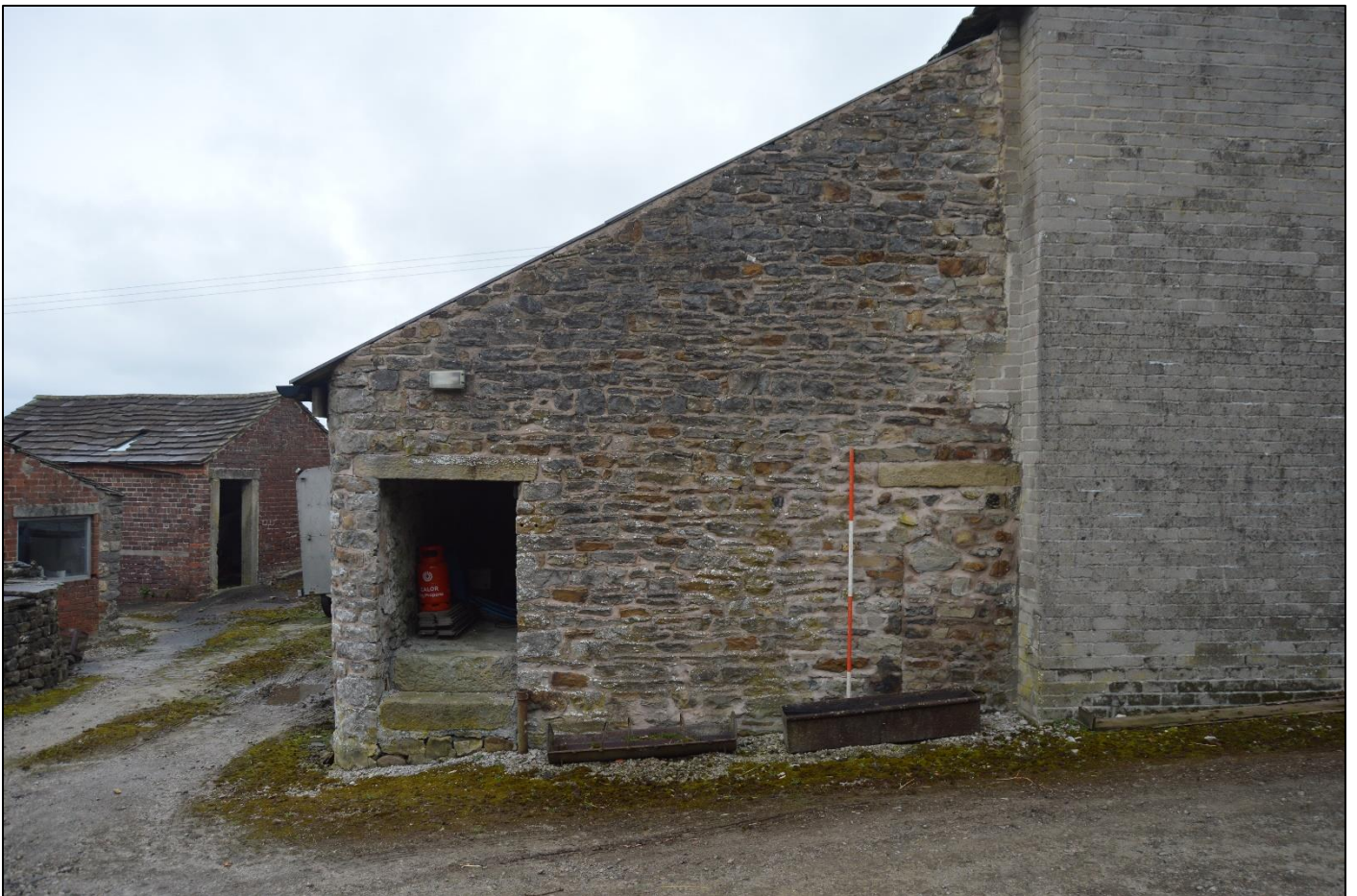
PL02: View of the north outshut from the west.
