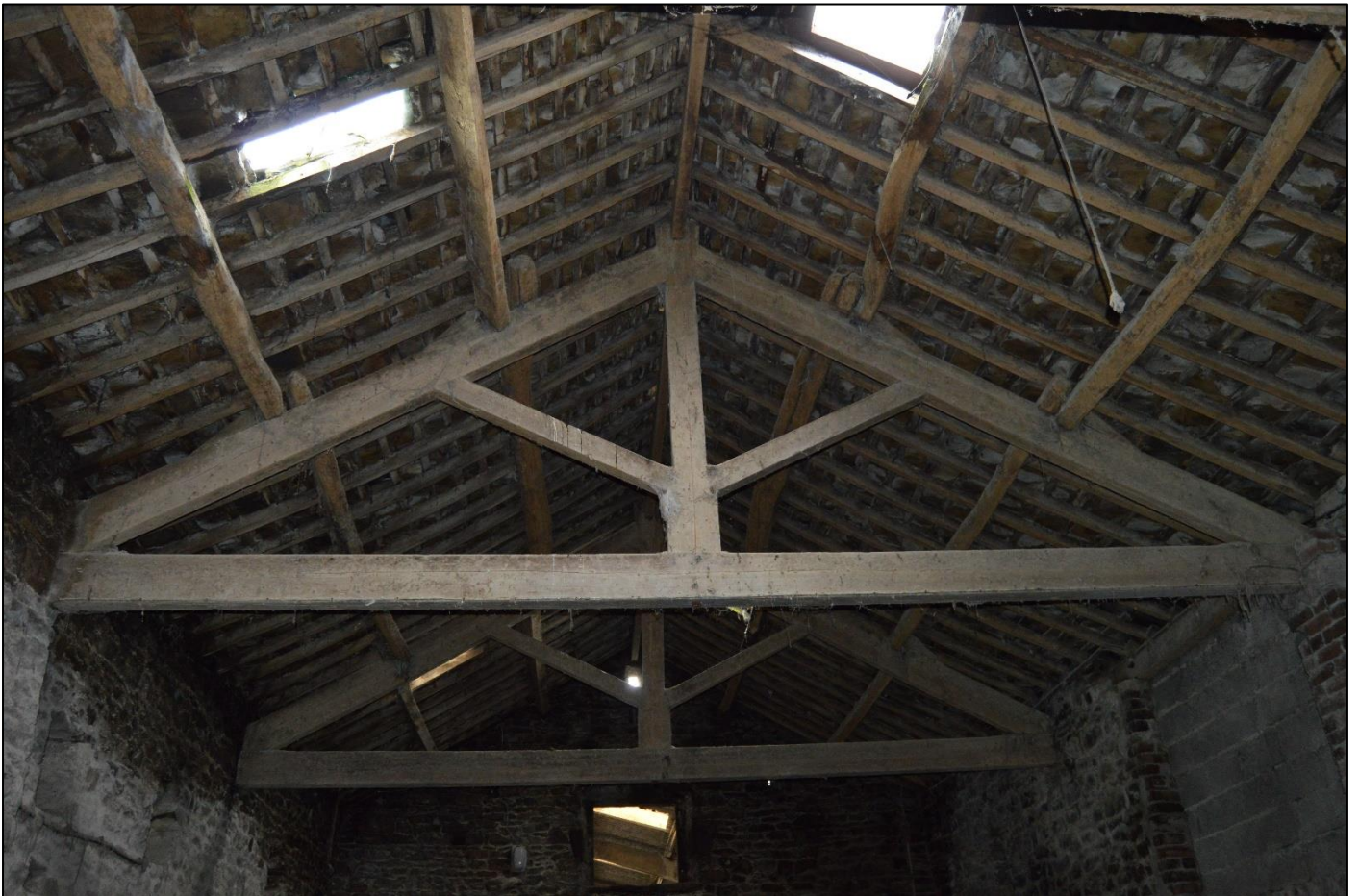
PL51: View of king post roof trusses over the east end of the original barn.
