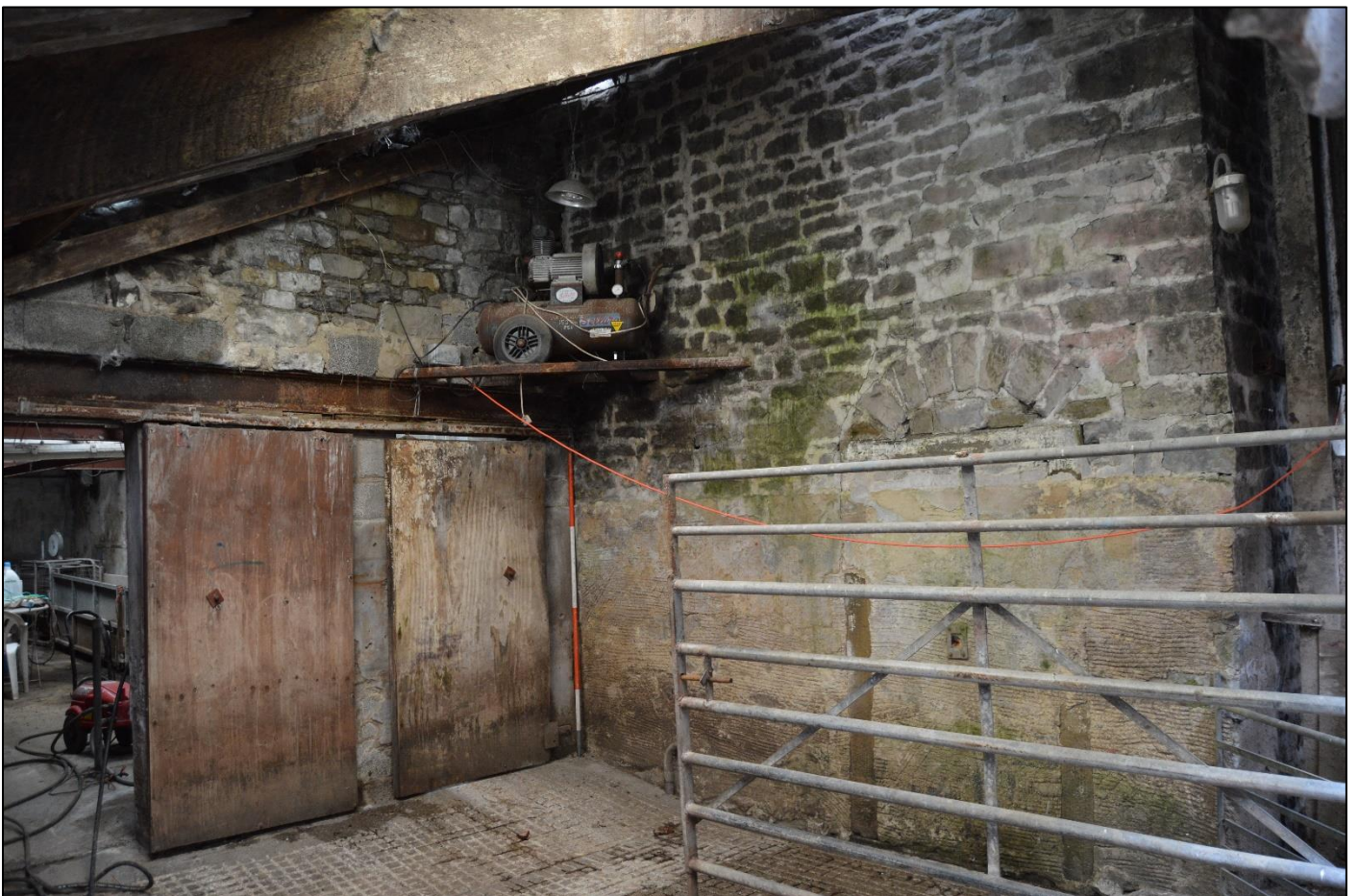
PL22: View of the south east corner of the barn. Note the blocked doorway to the south elevation.
