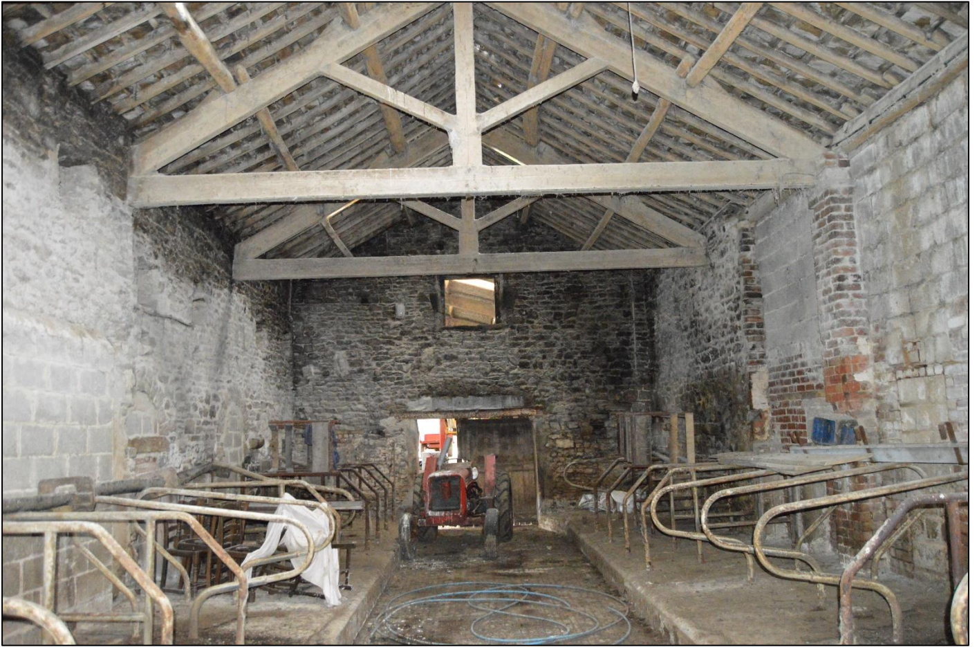
PL40: View east within the original barn.
