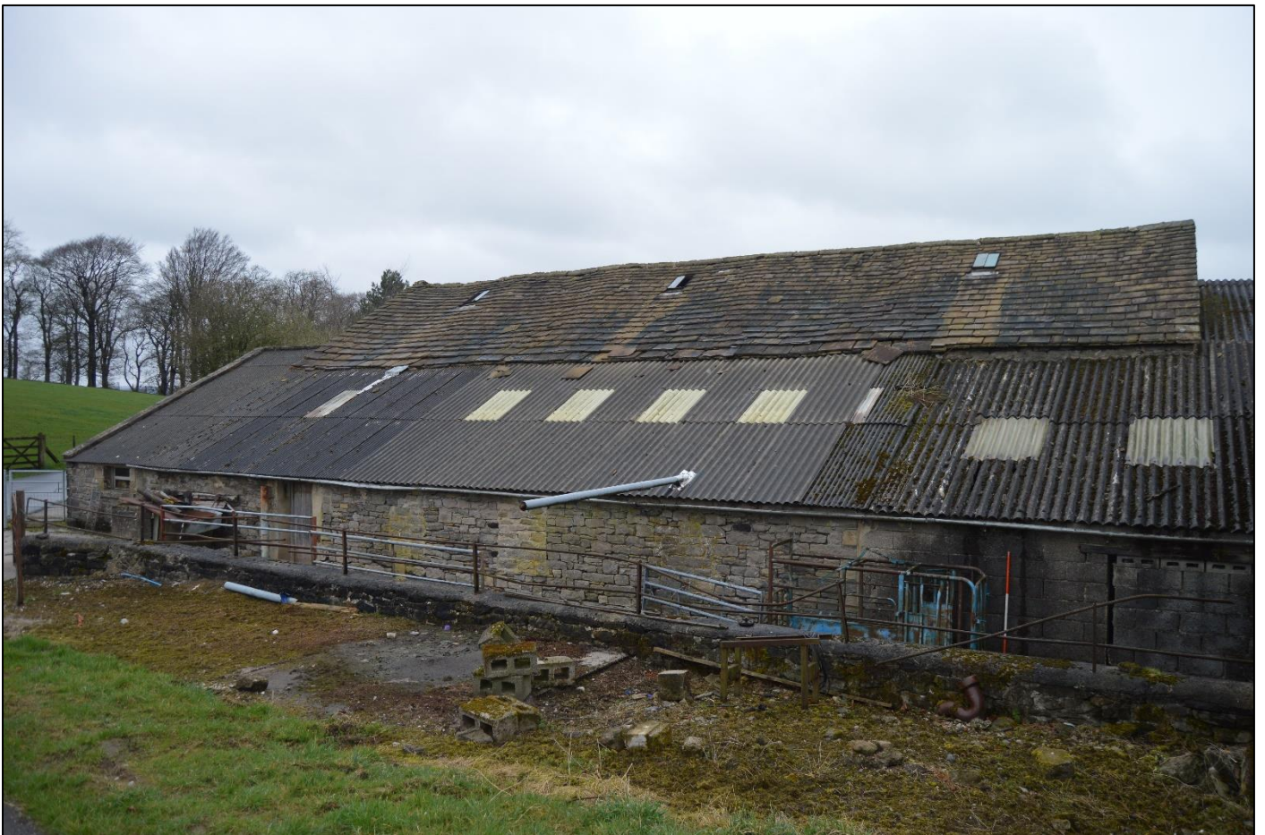
PL10: View of the barn from the south.
