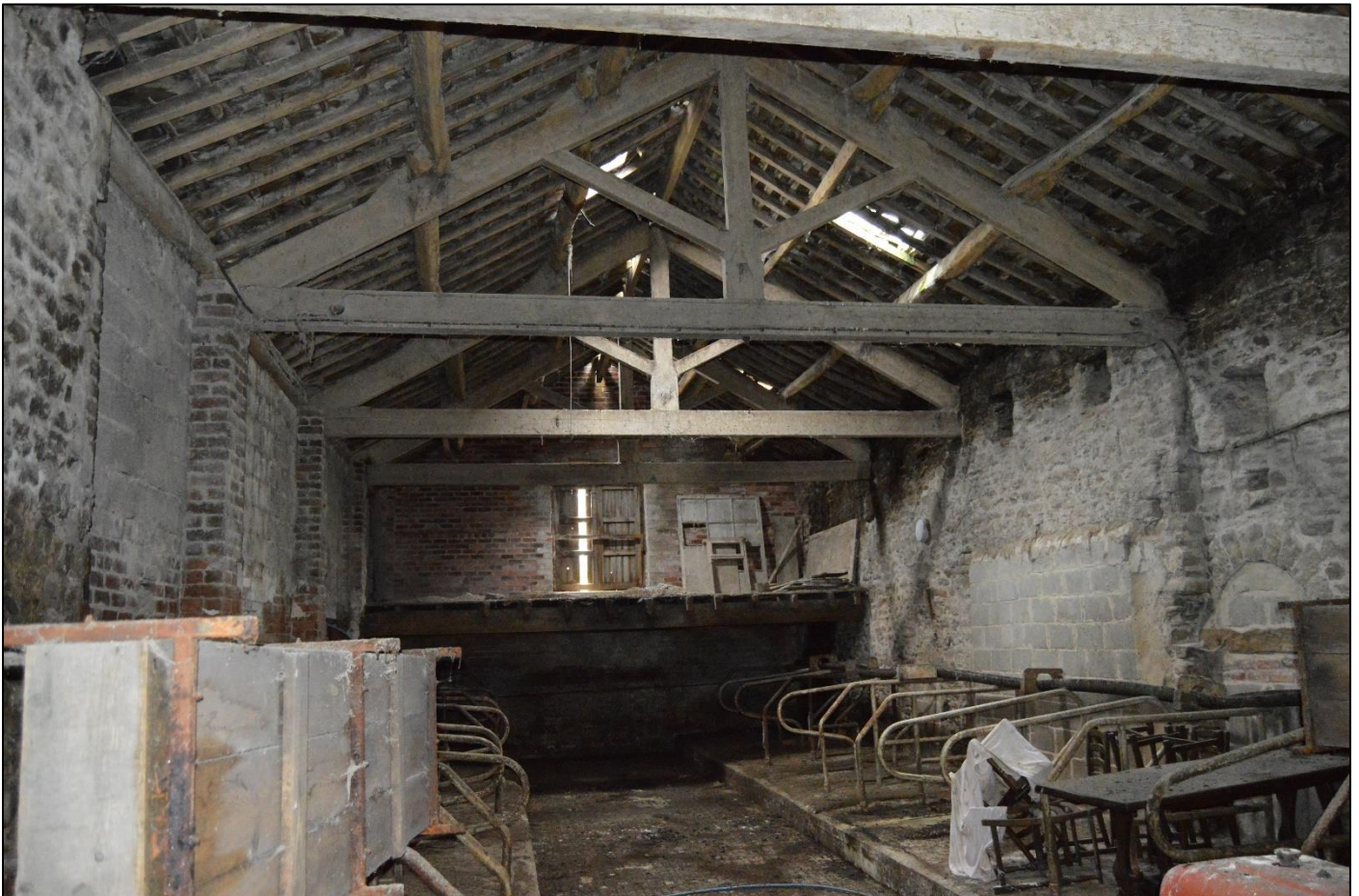
PL38: View west within the original barn.
