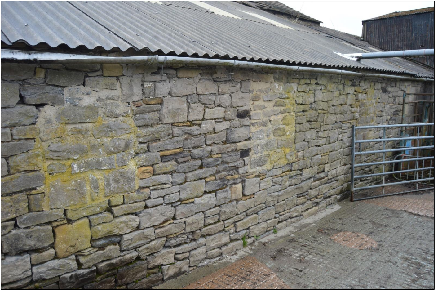
PL09: View of the 3no. blocked window openings to the south outshut.
