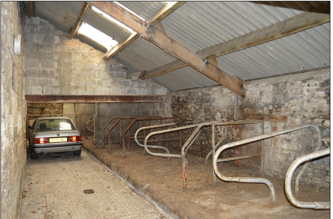
PL30: View west within the north outshut.
