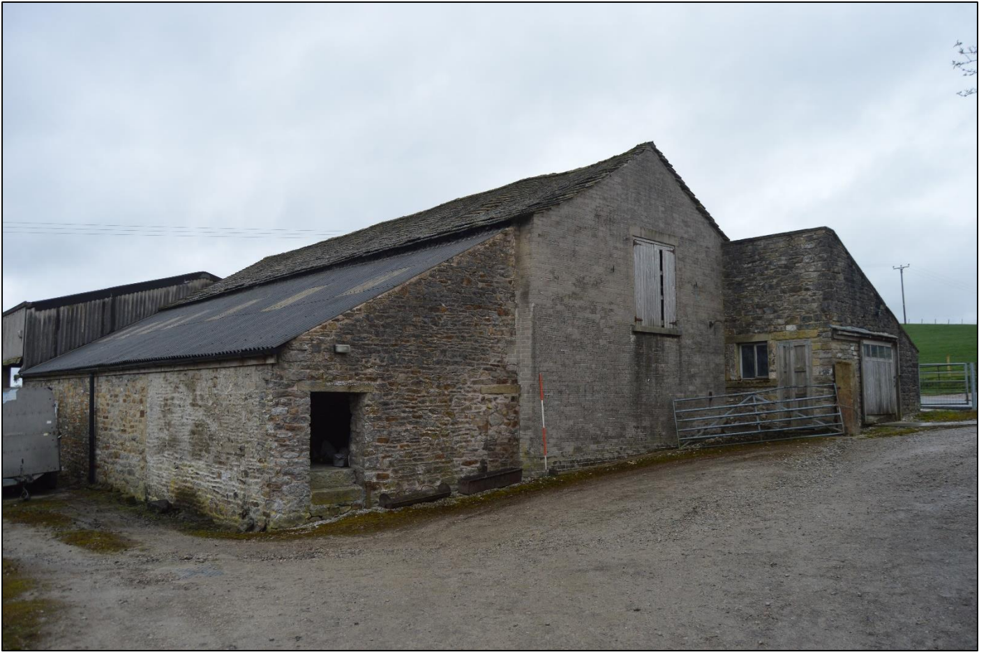
PL01: View of the barn from the west.
