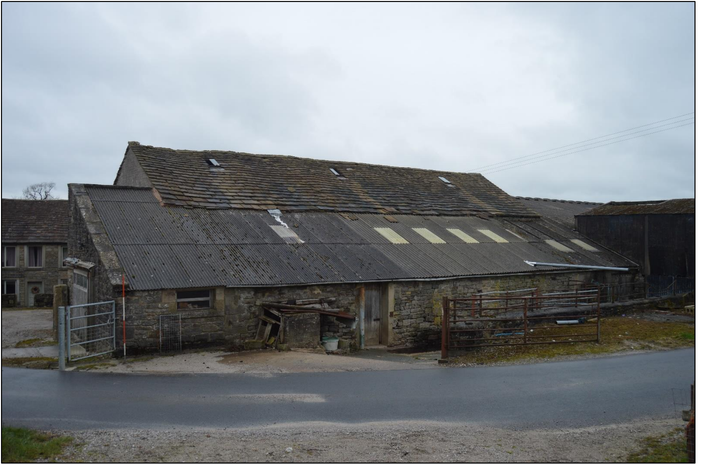
PL07: View of the barn from the south.
