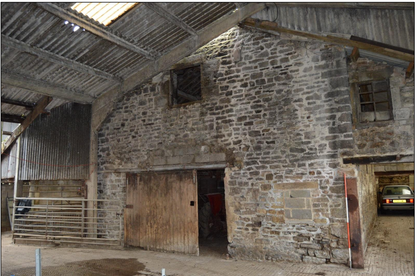
PL26: View of the east gable end elevation of the original barn.
