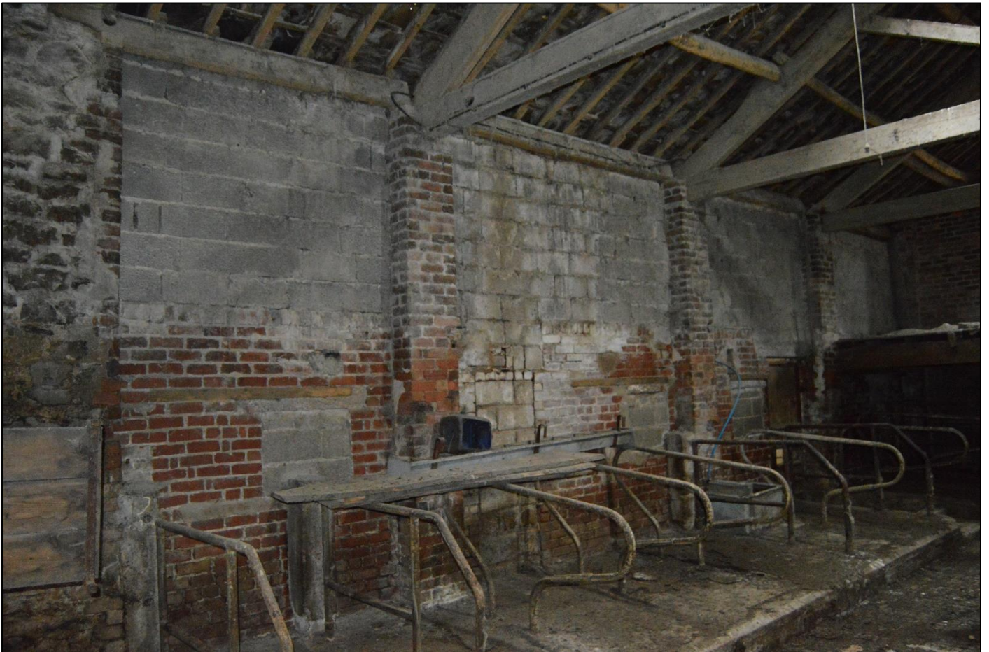
PL41: View of the phases of rebuilding of the west end of the south wall of the original barn.
