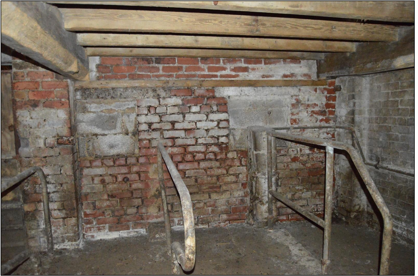
PL50: View south from below the west hay loft.
