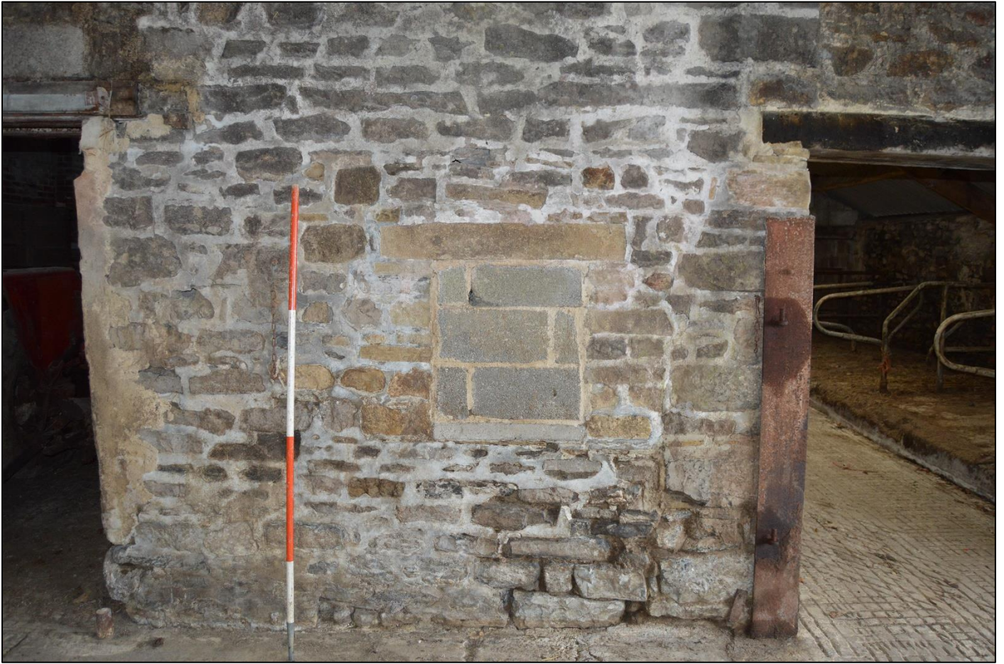
PL27: View of small blocked up window to the east gable end elevation of the original barn.
