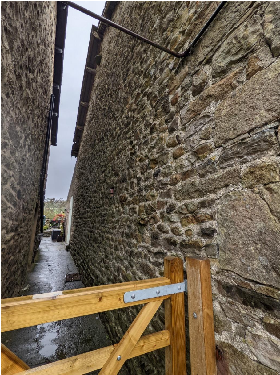
Gable Wall, adjacent to farmhouse, pointing in good condition
