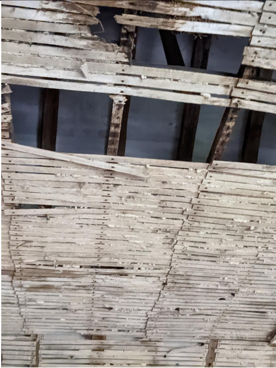
Roof space, showing modern breather membrane over rafters
