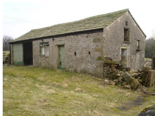
Southern Farm Building
