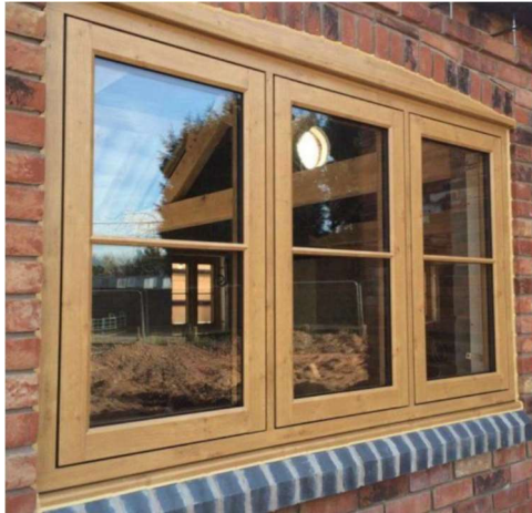
Appendix 4 Example of a flush finish timber window
