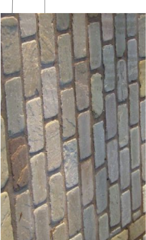
- Natural sandstone sets to entrance and to boarder of gravel.
