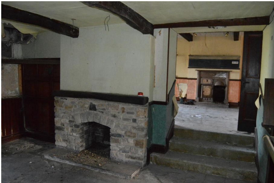
Snug –New wood burning stove to be installed.
