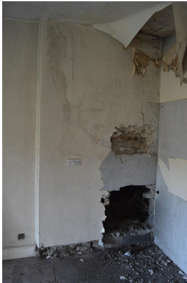
Master Bedroom – No surround present, to be retained and concealed.
