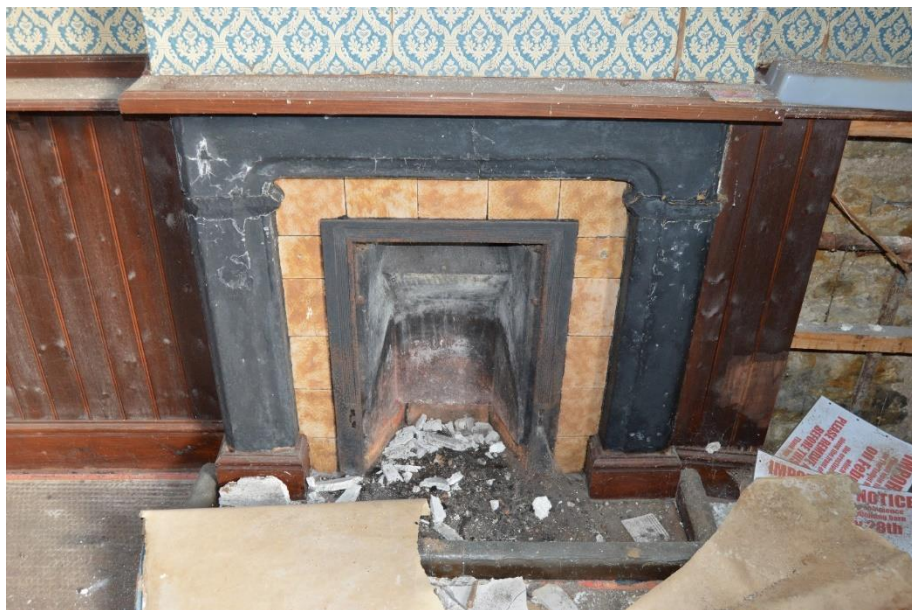
Kitchen – Surround to be retained and concealed within kitchen design.
