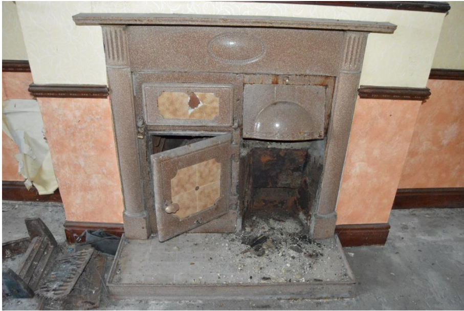
Games Room – To be carefully restored for decorative purposes.
