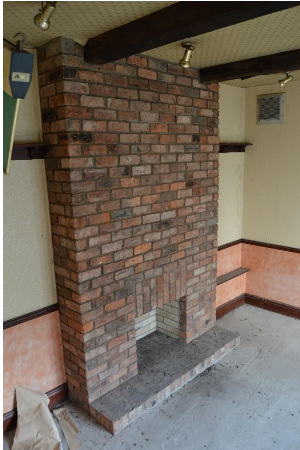
Living Room (Holiday Let) – New wood burning stove to be installed.
