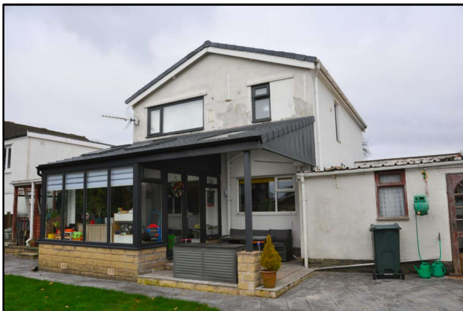
Image showing south (rear) elevation at 55 Edisford Road
