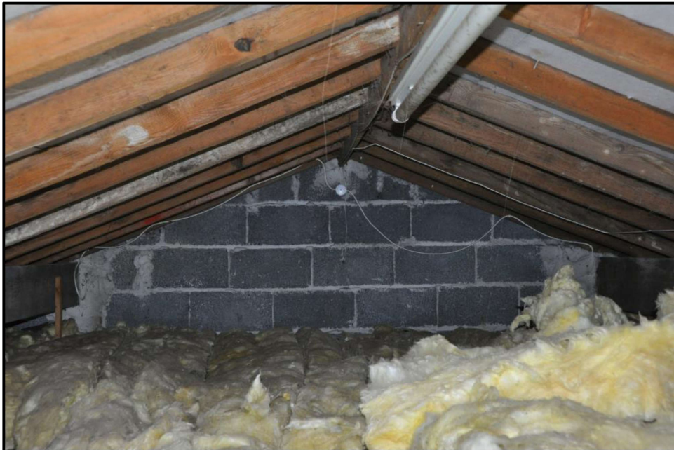
Image showing shallow roof void, no potential access points present
