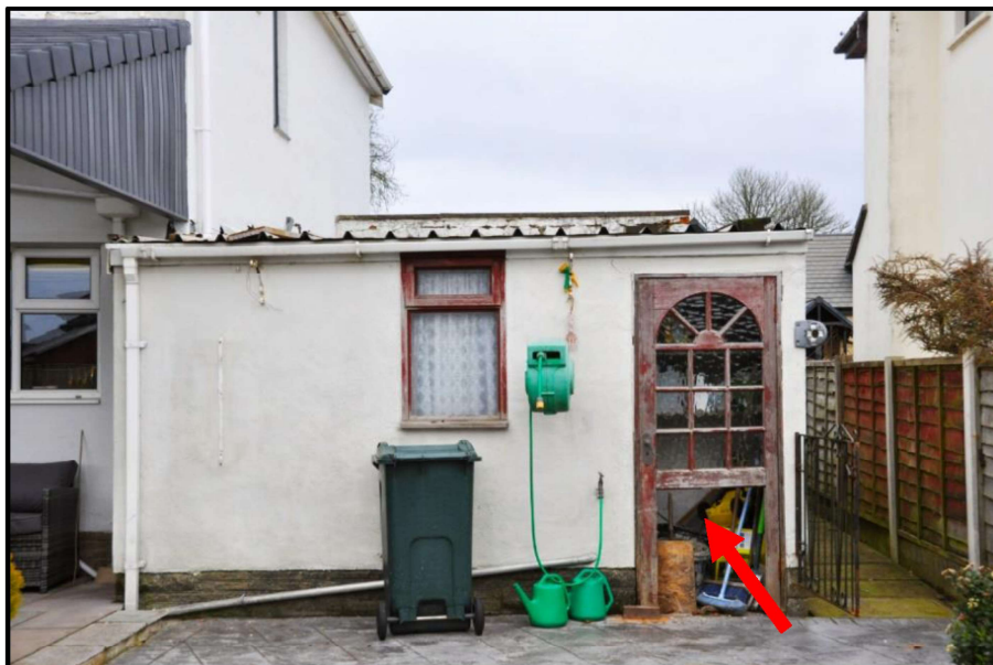
Image of garage storage room, showing potential access for use by nesting birds (red arrow)
