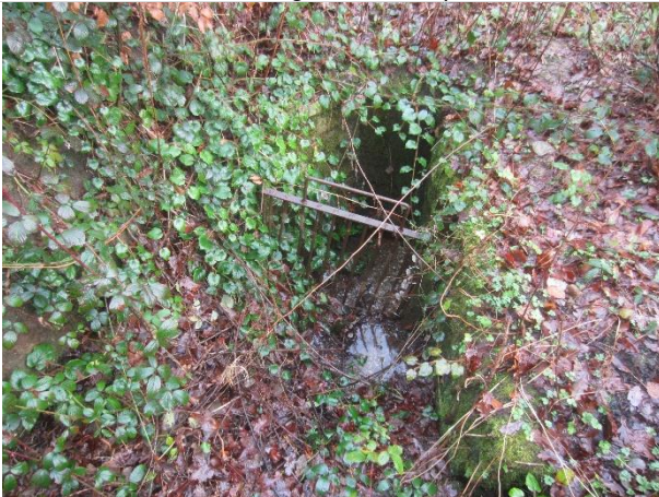
Photo 11: Drain enters a pipe that carries water beneath the driveway to the east
