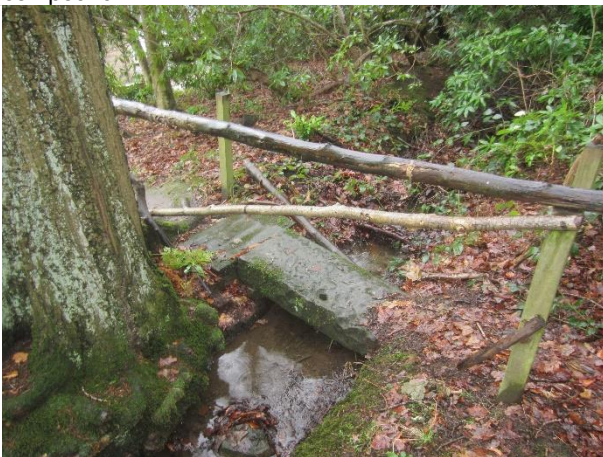
Photo 9: Stone slab bridge over the ephemeral drain
