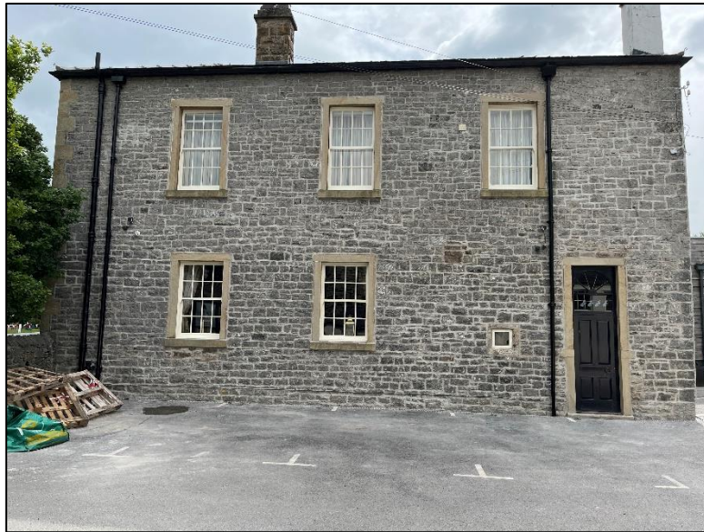
Fig. 2 west elevation following render removal and re-pointing which is now reflective of the North (front) elevation with exposed quoins and window surrounds.
