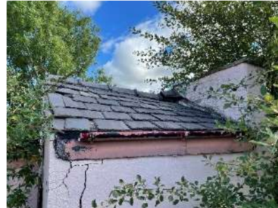
B2 Gaps around and behind guttering
