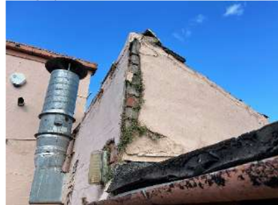
B4 gaps around bricks and render
