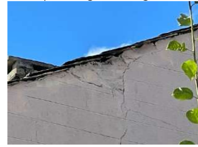
B2 gaps behind guttering
