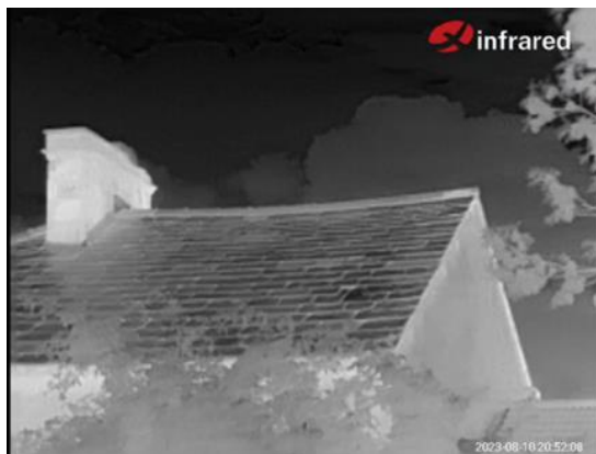
Figure 2 Thermal image taken during the survey showing the northeastern elevation, viewed from the east
