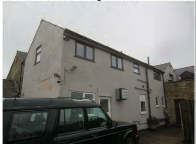
Photo 18: Building 1 section 1c (northern and western elevations)
