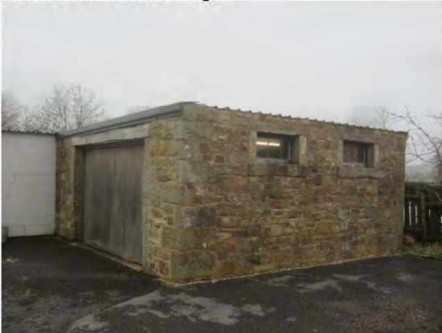
Photo 27: Western and southern elevations of Building 4
