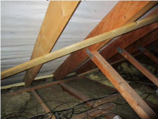
Photo 21: Roof void at Building 1 section 1d
