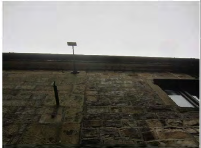
Photo 12: Tight fitting timber fascia at southern elevation of Building 1 section 1a
