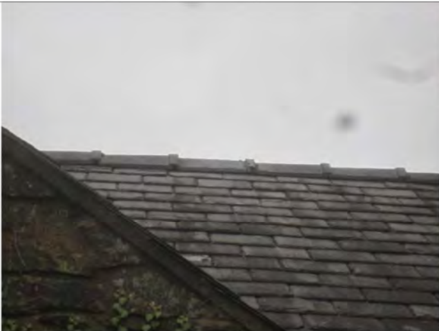
Photo 13: Ridge copings at Building 1 section 1a
