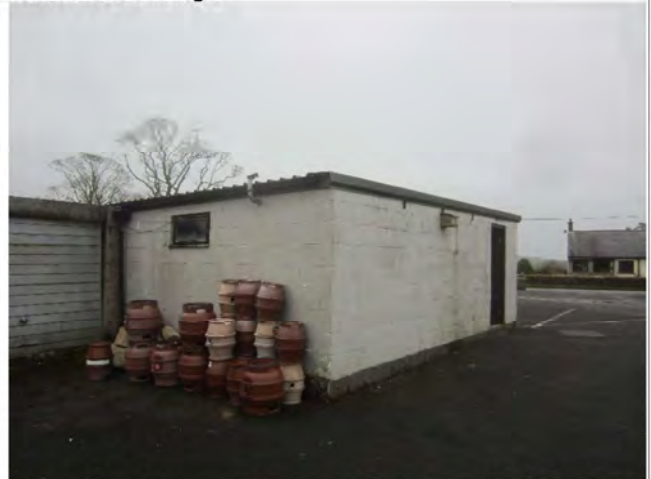
Photo 28: Northern and western elevations of Building 4
