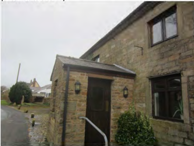
Photo 11: Porch attached to Building 1 section 1a
