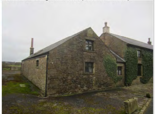
Photo 22: Western and southern elevations of Building 5
