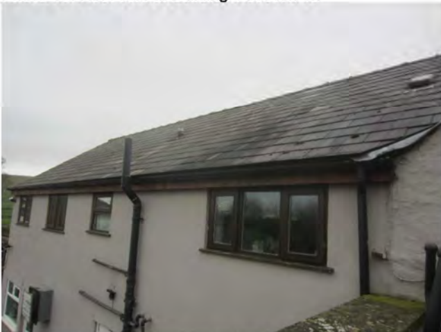
Photo 17: Building 1 section 1c (northern elevation)
