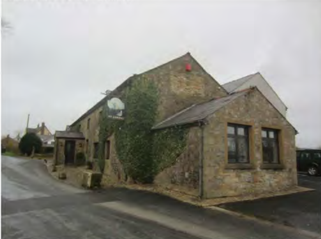
Photo 9: Southern and eastern elevations of Building 1 (sections 1a and 1b)
