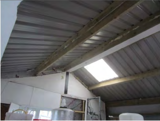
Photo 25: Interior of Building 2
