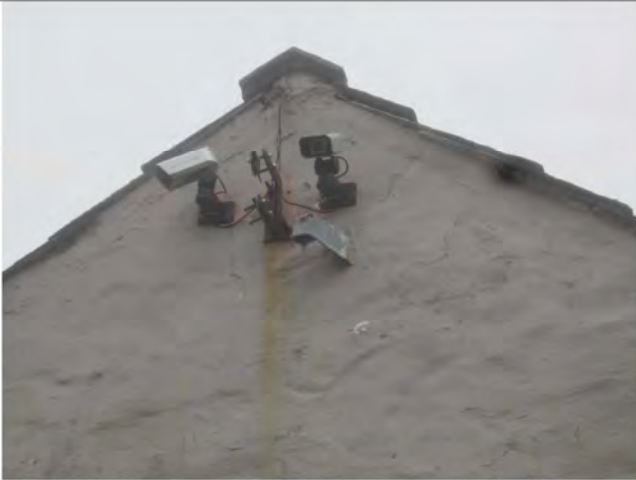
Photo 19: Building 1 section 1c (northern elevation)
