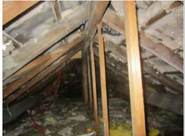
Photo 16: Roof void at Building 1 section 1a
