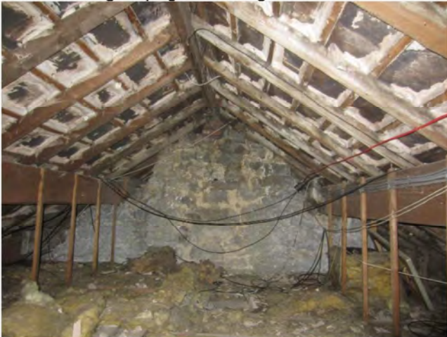
Photo 15: Roof void at Building 1 section 1a
