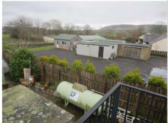
Photo 4: Asphalt covered hard-standing and Buildings 2 to 4
