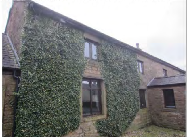
Photo 10: Southern elevation of Building 1 section 1a
