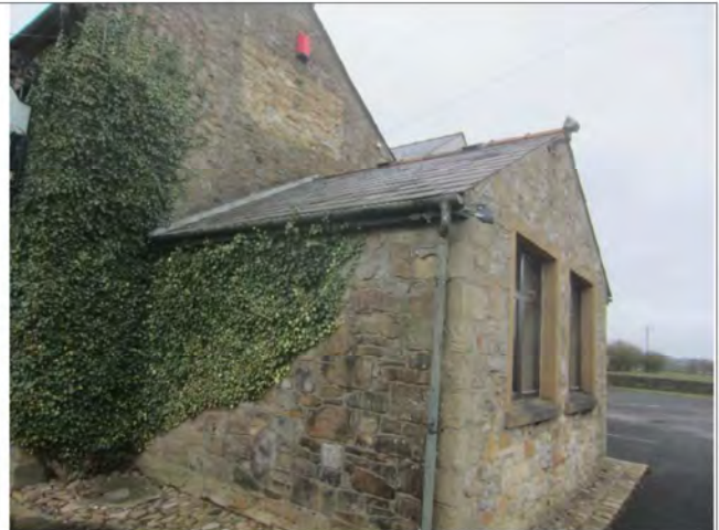
Photo 14: Building 1 section 1b
