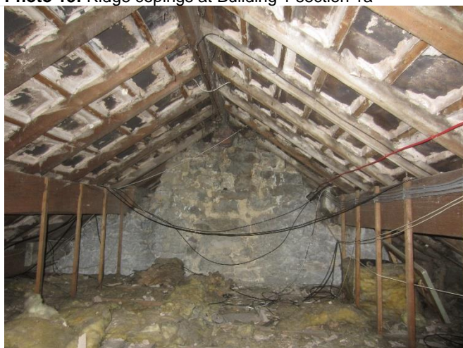
Photo 15: Roof void at Building 1 section 1a
