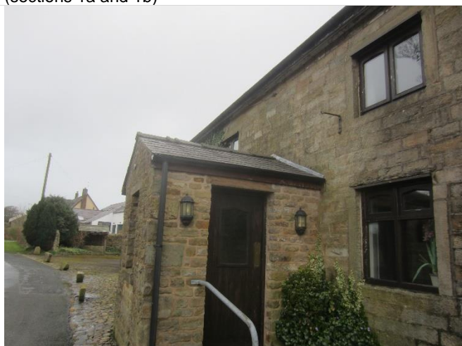
Photo 11: Porch attached to Building 1 section 1a
