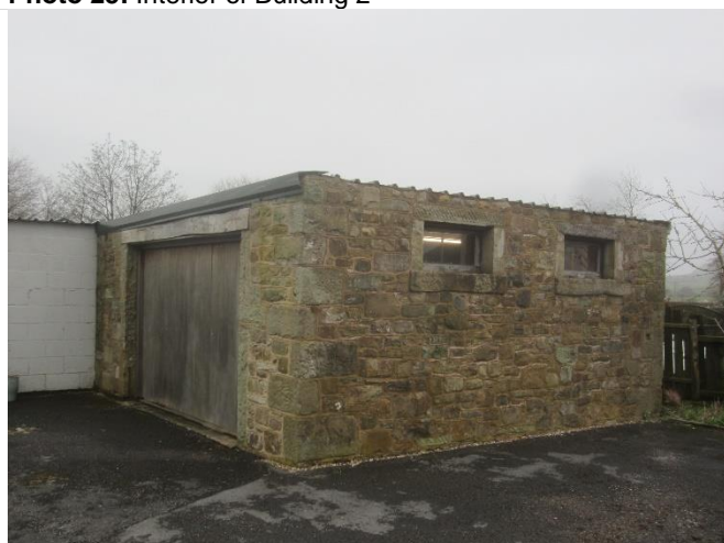
Photo 27: Western and southern elevations of Building 4
