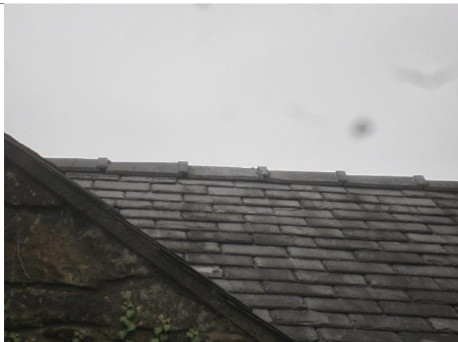
Photo 13: Ridge copings at Building 1 section 1a
