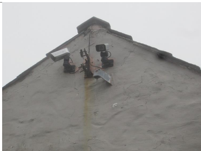
Photo 19: Building 1 section 1c (northern elevation)
