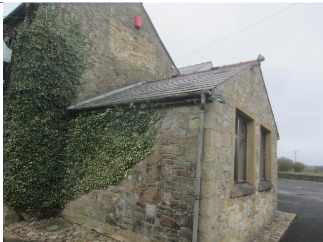
Photo 14: Building 1 section 1b
