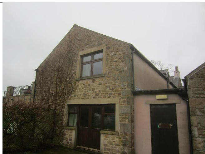
Photo 20: Building 1 section 1d (northern elevation)
