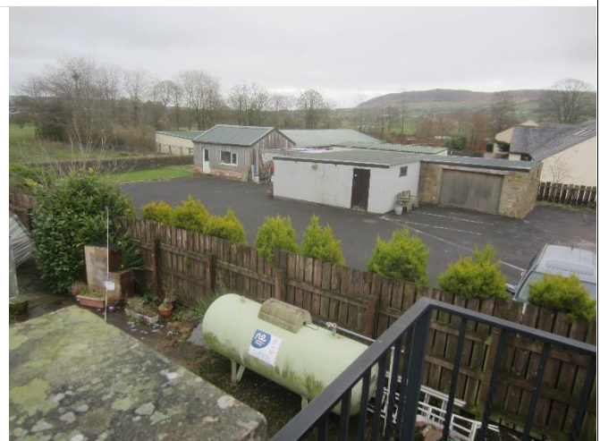
Photo 4: Asphalt covered hard-standing and Buildings 2 to 4
