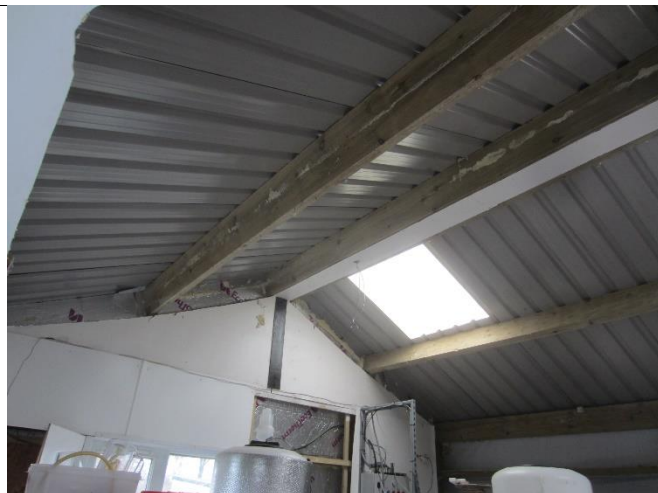
Photo 25: Interior of Building 2
