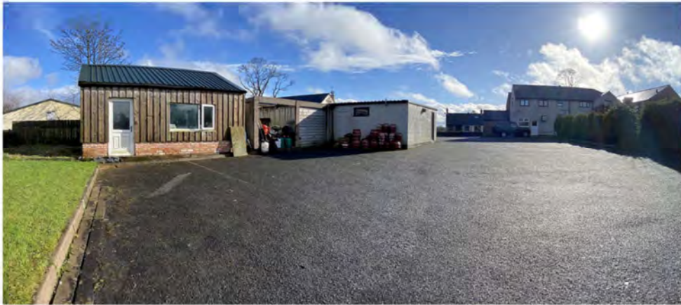
Looking Southeast Across The Car Park
