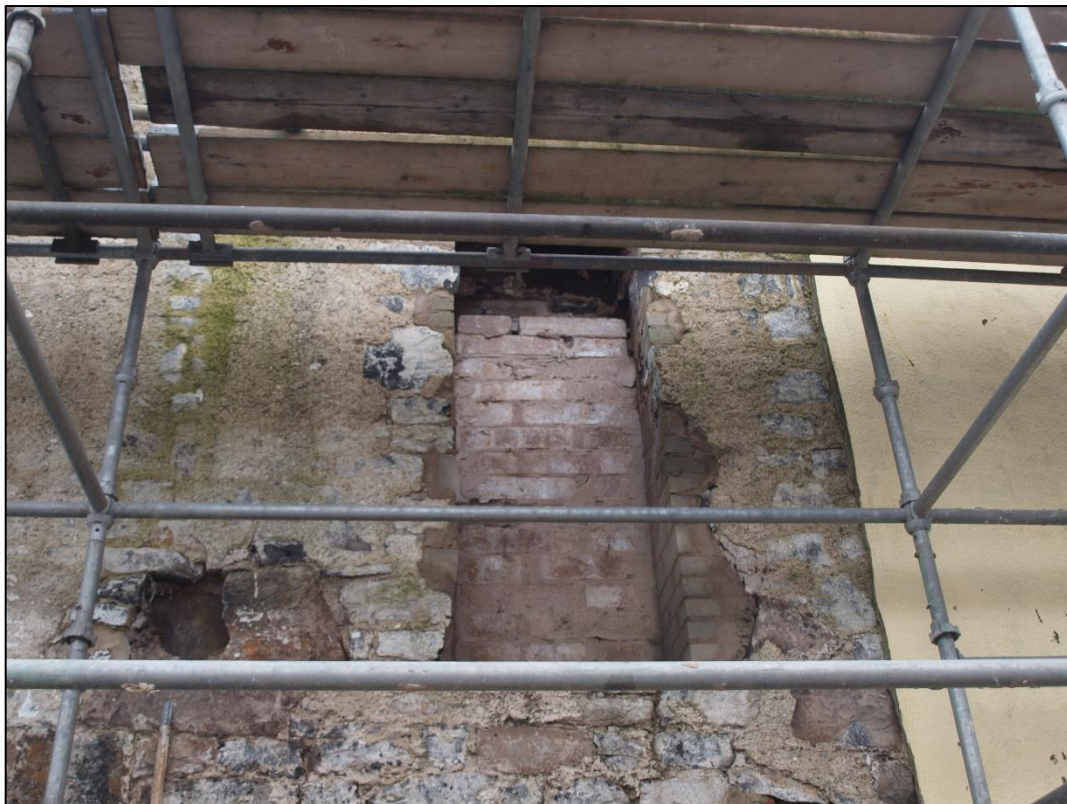
Plate 10: First floor inserted and blocked doorway
