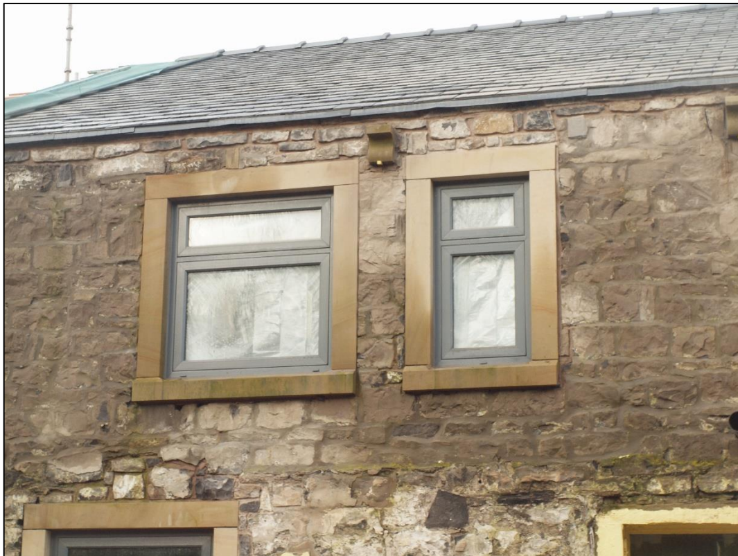
Plate 13: First floor windows to south end of east elevation
