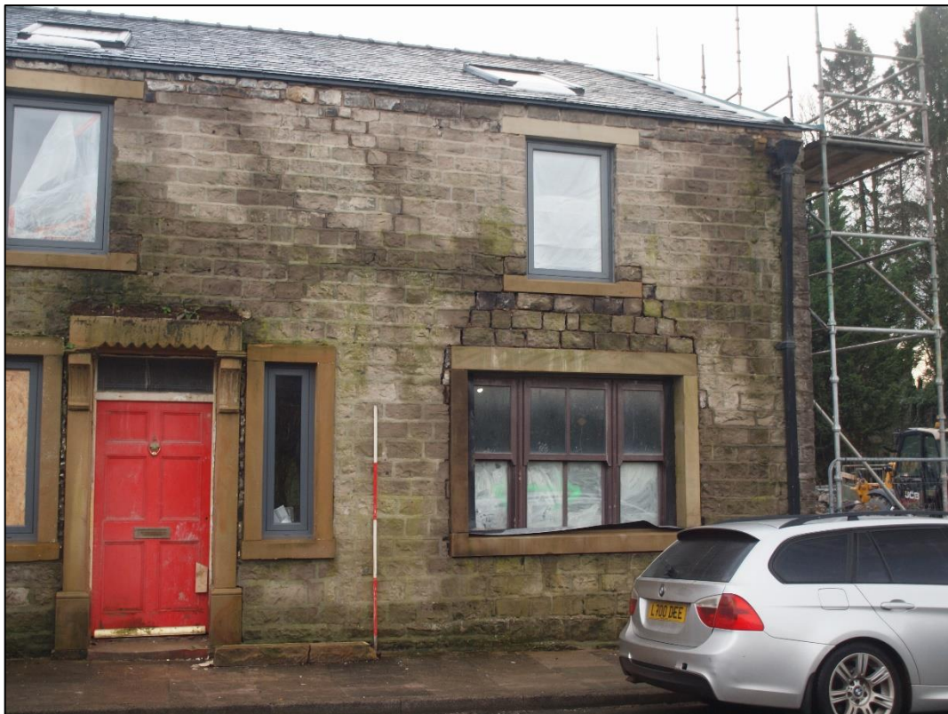
Plate 2: West elevation, south end
