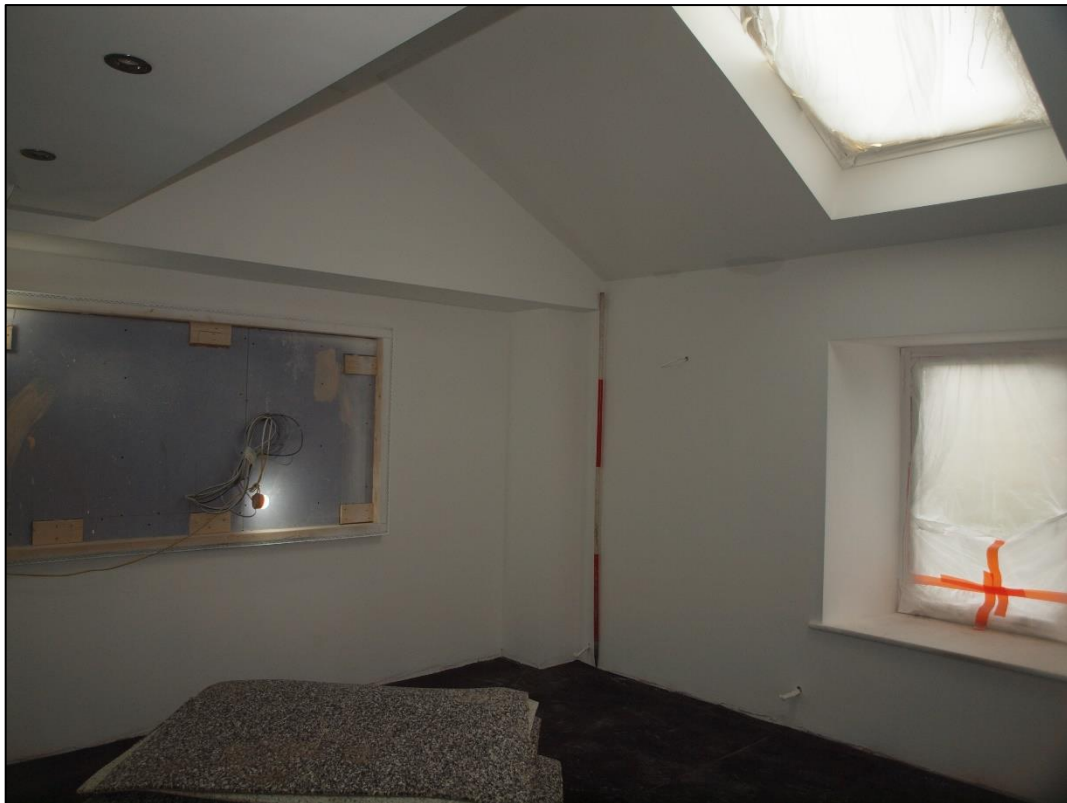
Plate 47: First floor northwest room
