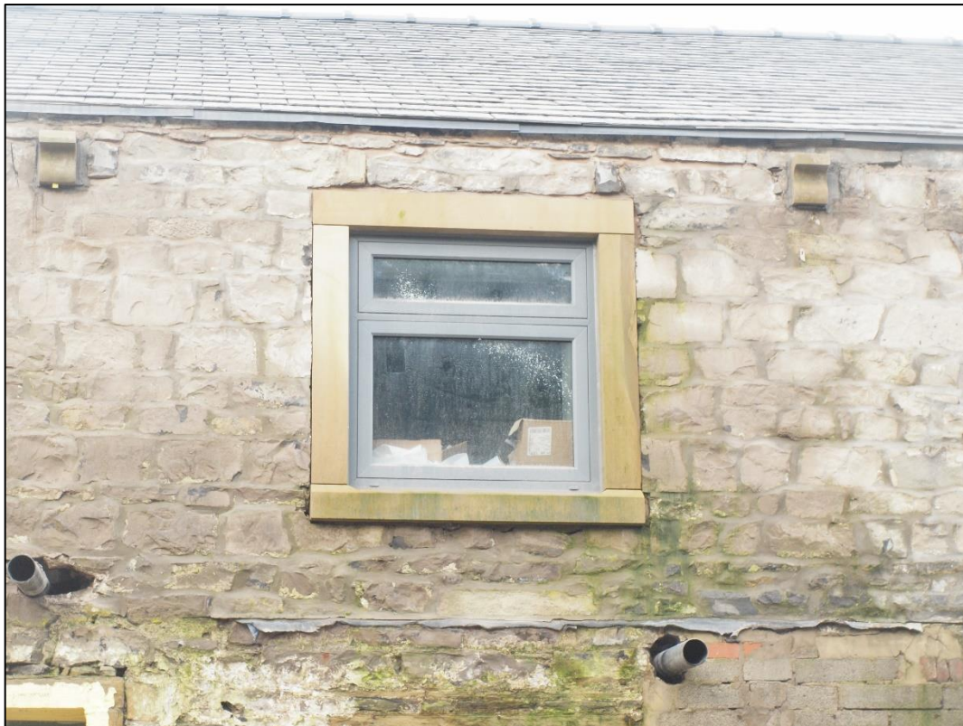
Plate 15: Central first floor window
