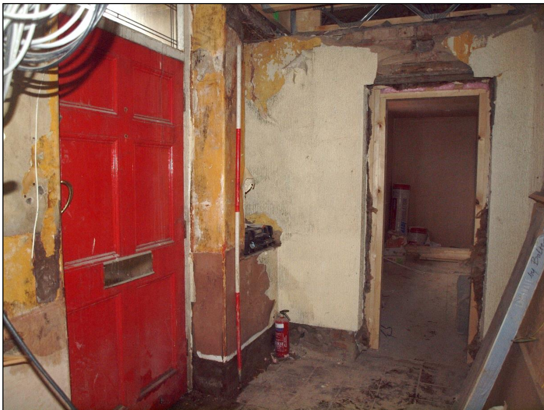
Plate 23: Ground floor entrance lobby showing main doorway to the left
