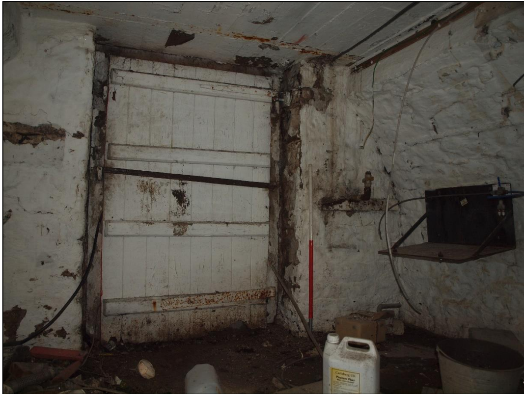
Plate 39: Southern room of cellar showing door in western wall
