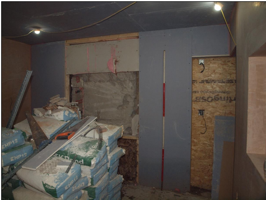
Plate 26: Northern room eastern end showing blocked openings
