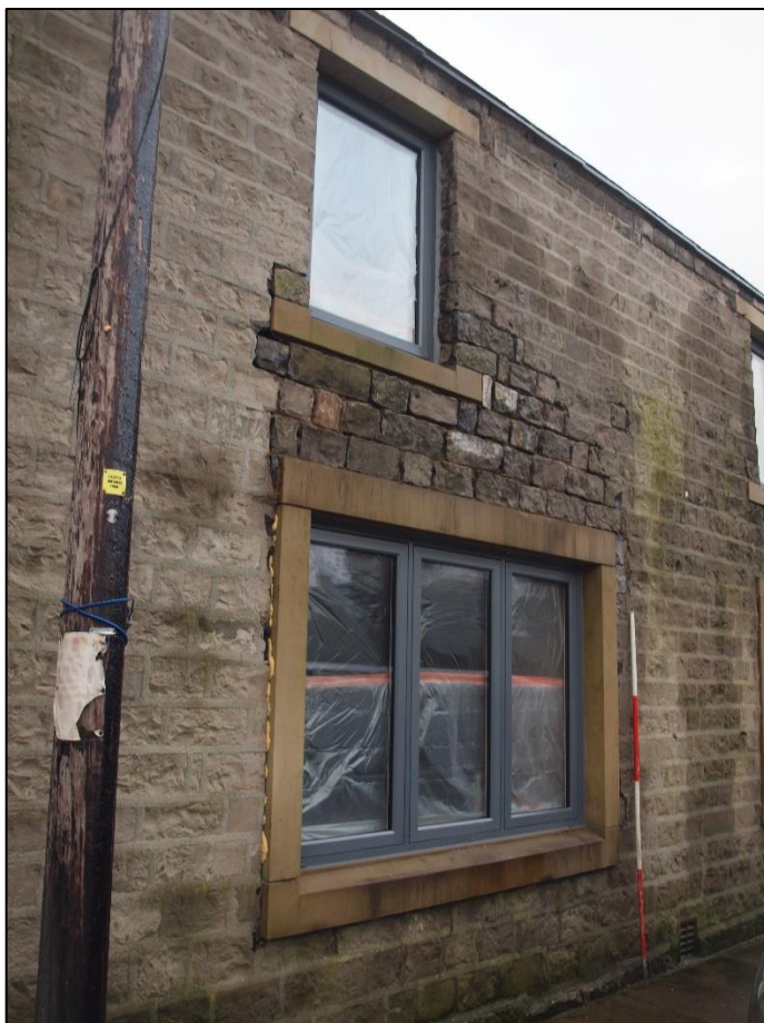
Plate 6: Rebuilding between ground and first floor windows
