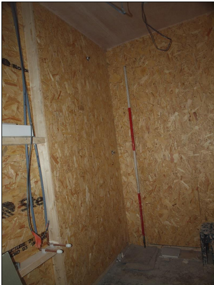
Plate 28: Boarded out room
