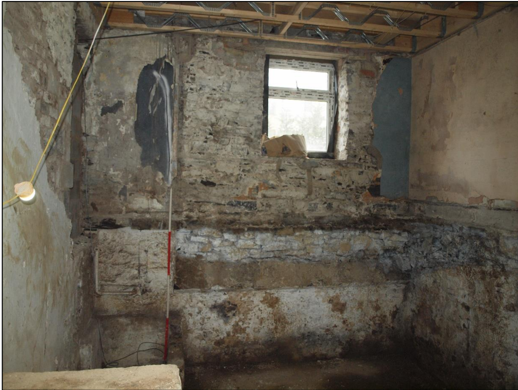
Plate 31: Southern end showing void to cellar looking east
