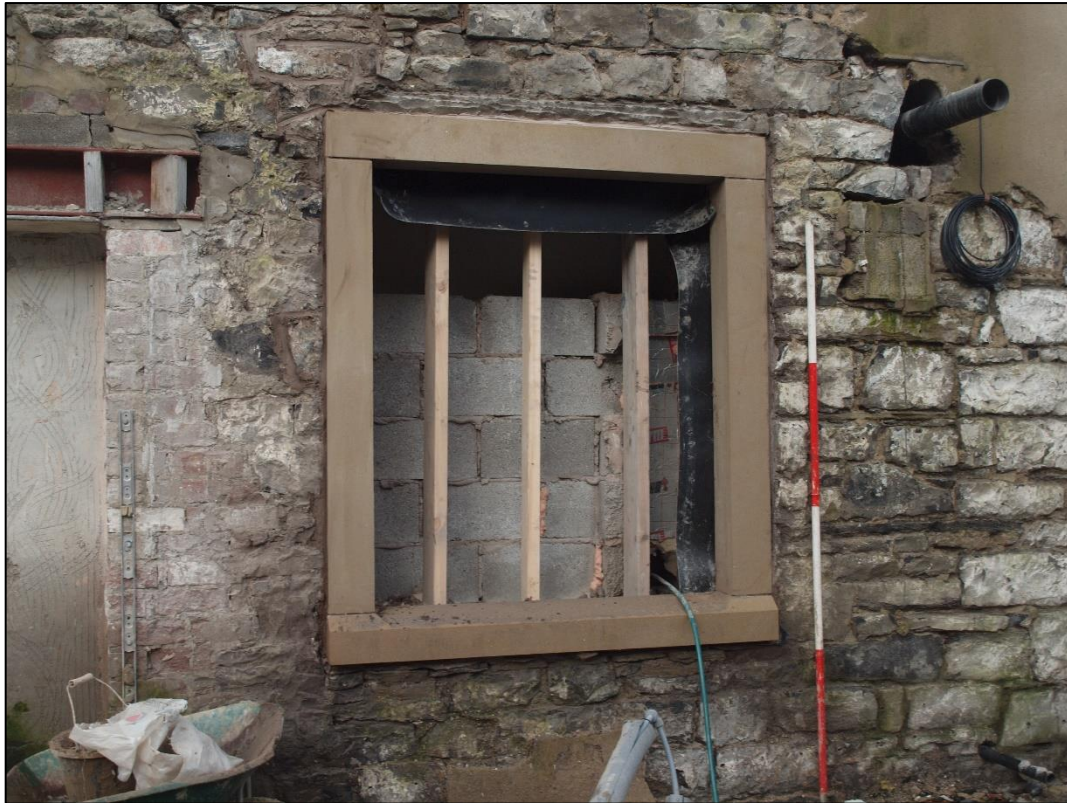
Plate 21: Ground floor window showing internal blocking
