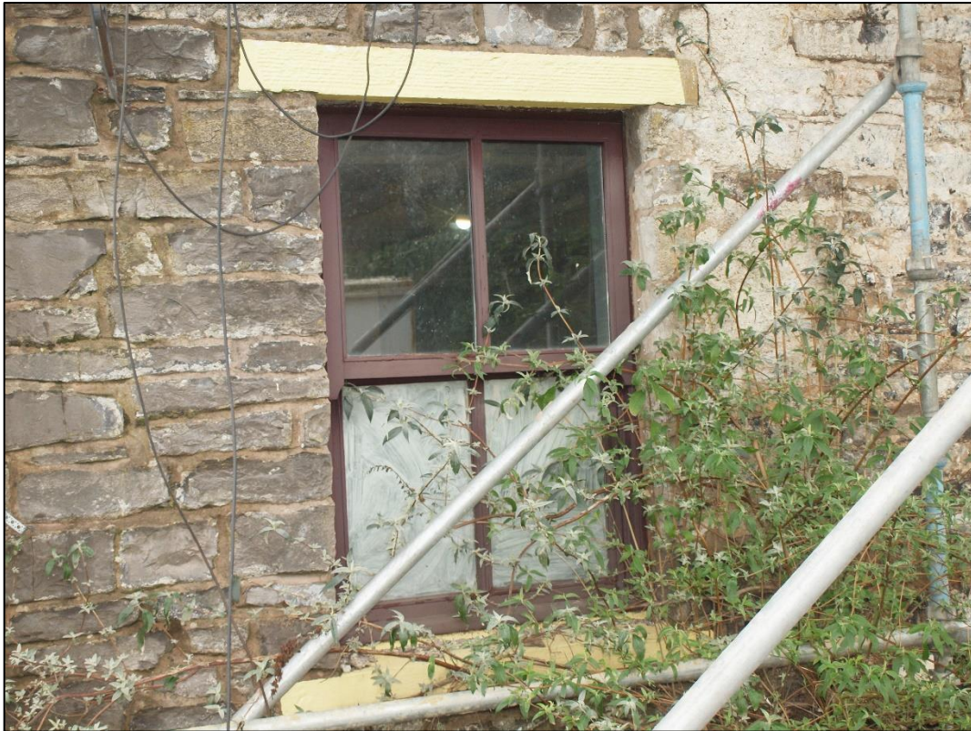
Plate 11: Ground floor window to west side of southern gable
