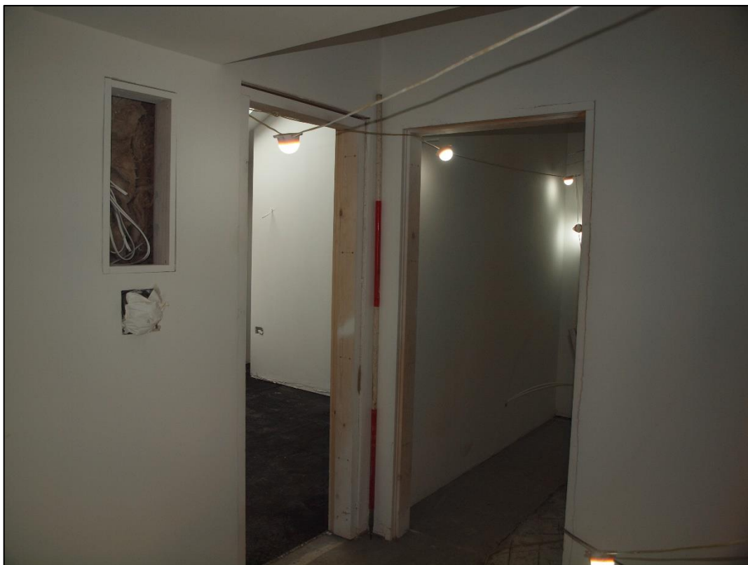
Plate 44: First floor corridor looking north
