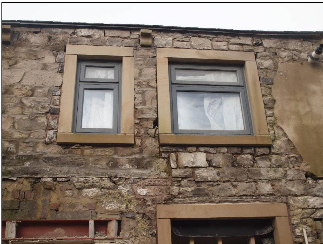
Plate 14: First floor windows to north end of east elevation
