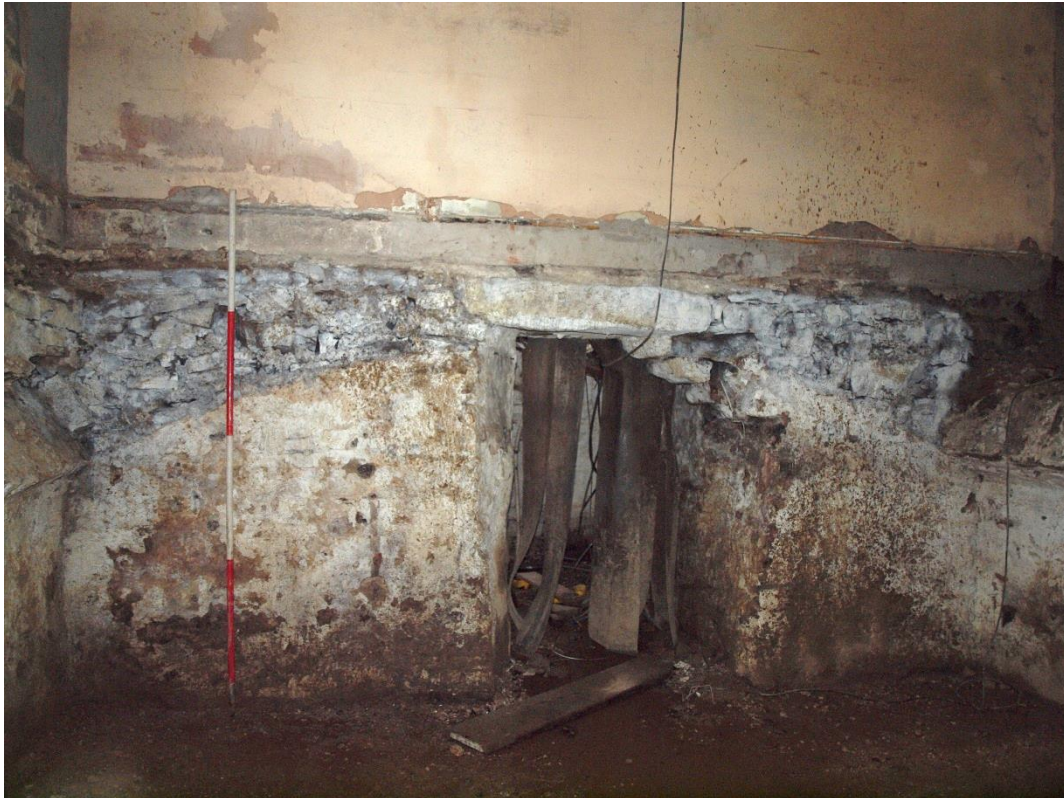
Plate 35: Southern wall of cellar showing doorway and scar of former arch with scar of removed ground floor level above
