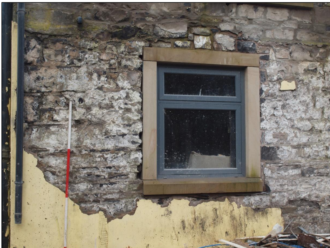
Plate 16: Ground floor window at southern end of east elevation
