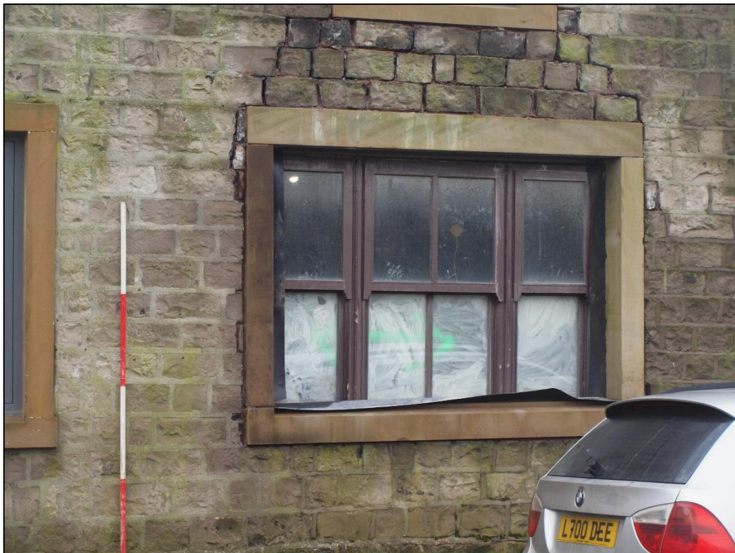
Plate 4: Southern window in west elevation
