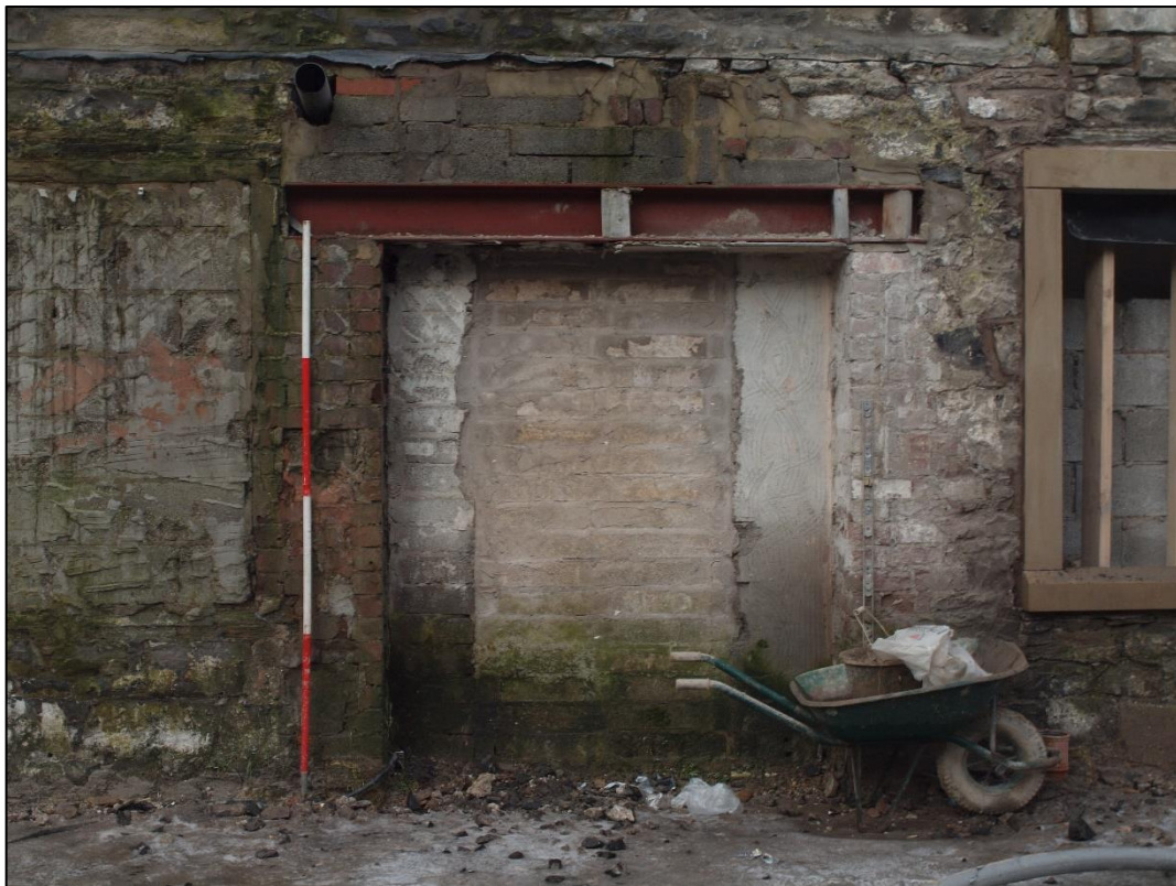
Plate 20: Inserted and blocked loading bay opening with blocked personnel doorway within it
