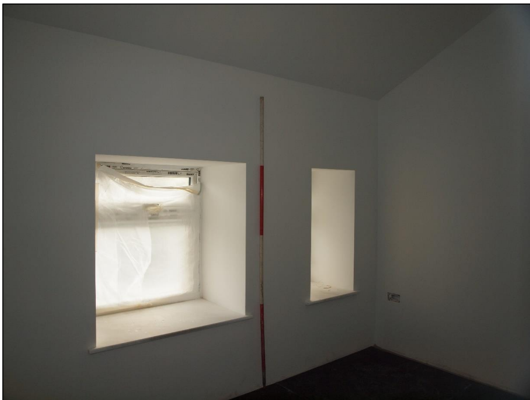
Plate 48: First floor northeast room
