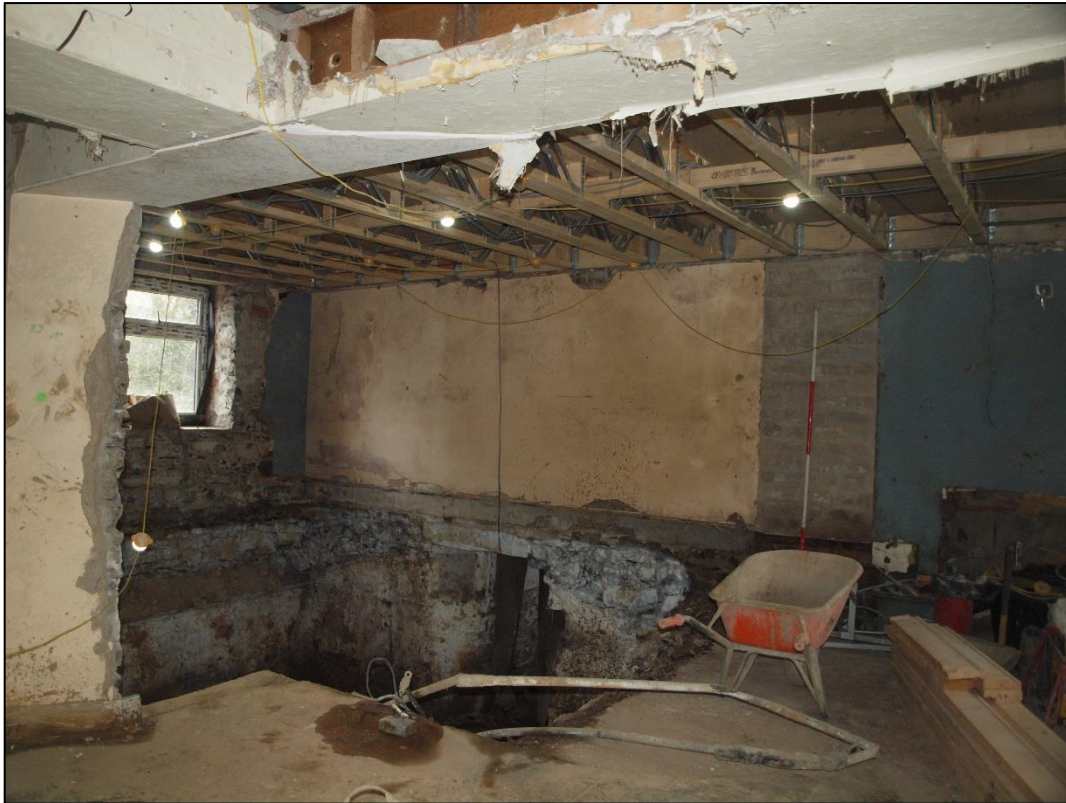
Plate 29: Ground floor southern room looking south
