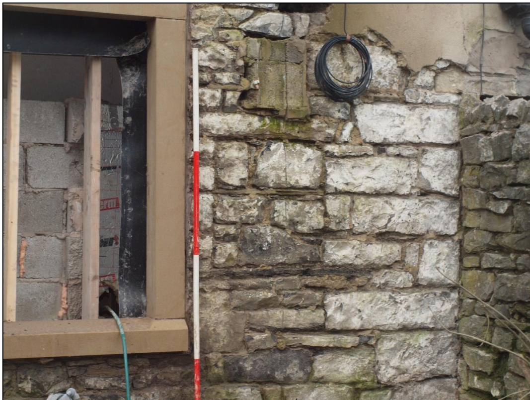
Plate 22: Small blocked window at north end of elevation, blocked with stone
