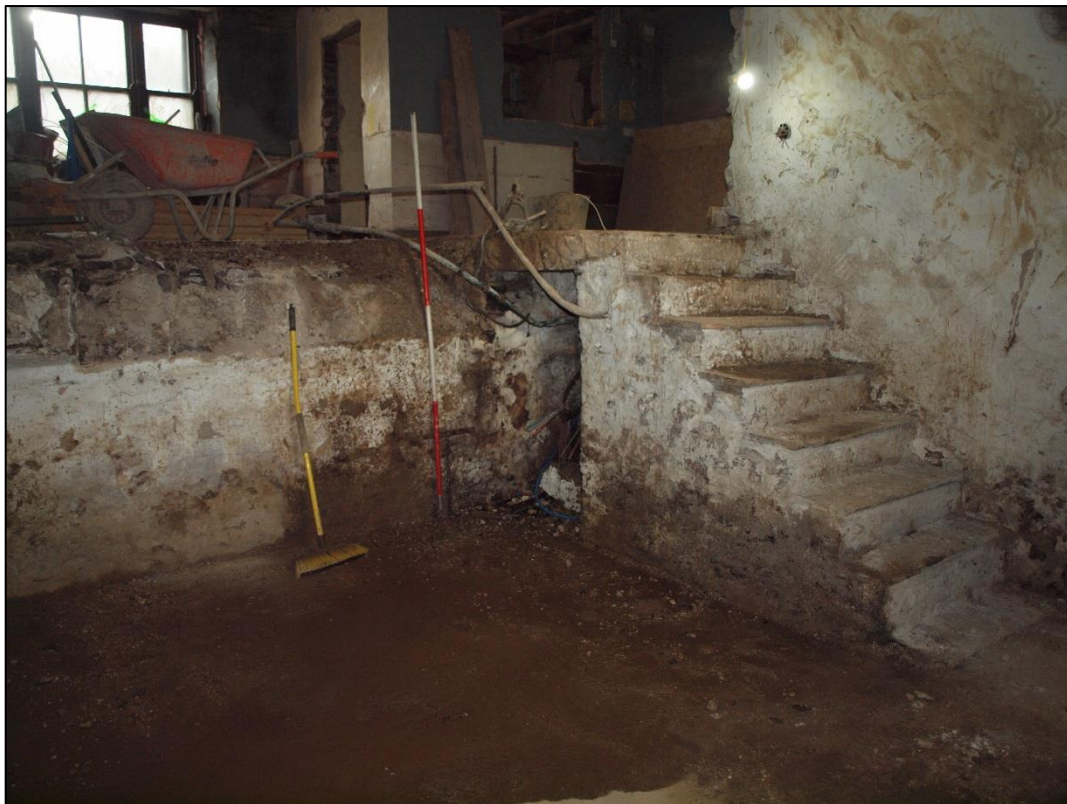
Plate 38: Cellar showing staircase to northwest corner
