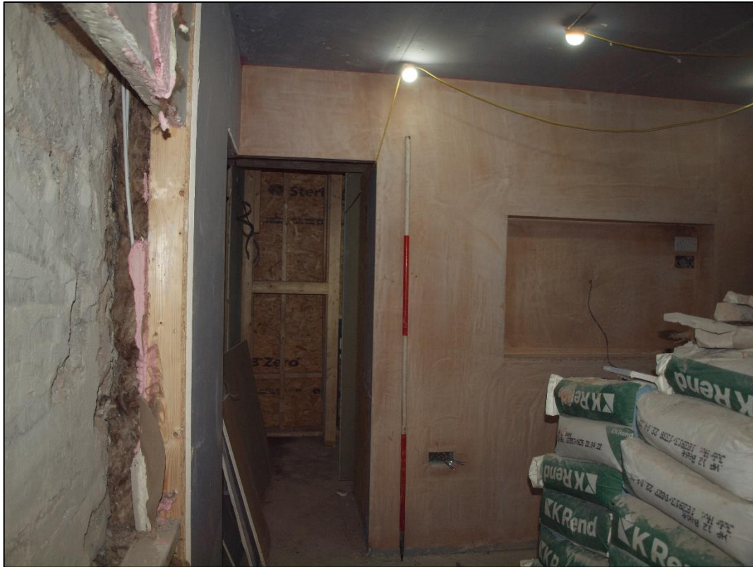
Plate 27: Modern stud walls to the south of room above
