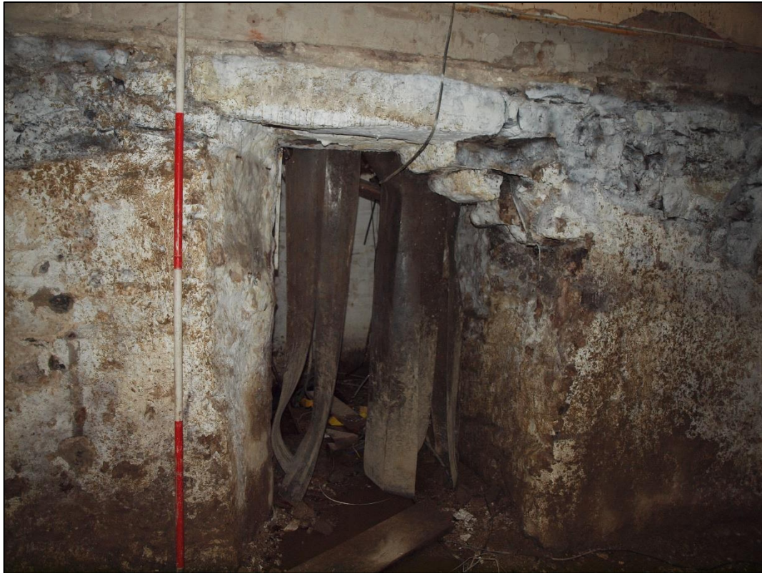
Plate 37: Detail of doorway
