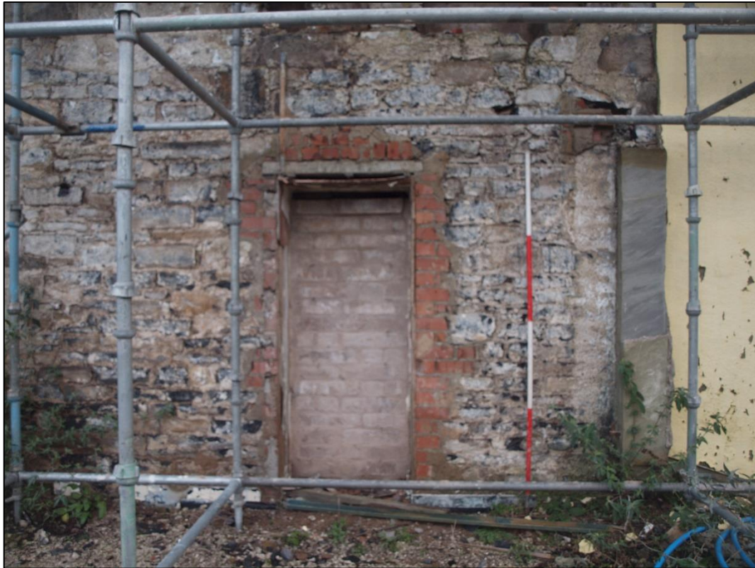
Plate 9: Ground floor of gable showing inserted and then blocked doorway
