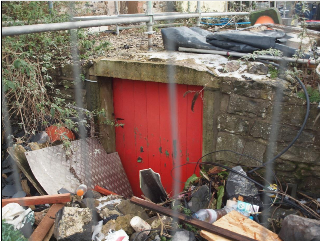
Plate 7: Cellar entrance to south side of west elevation
