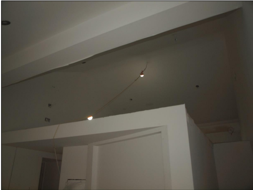
Plate 49: Room above showing plastered roof
