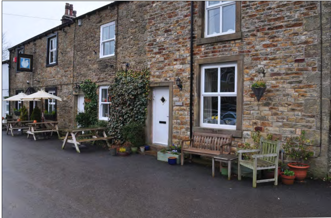
Photo 2: Street frontage, with adjoining houses
