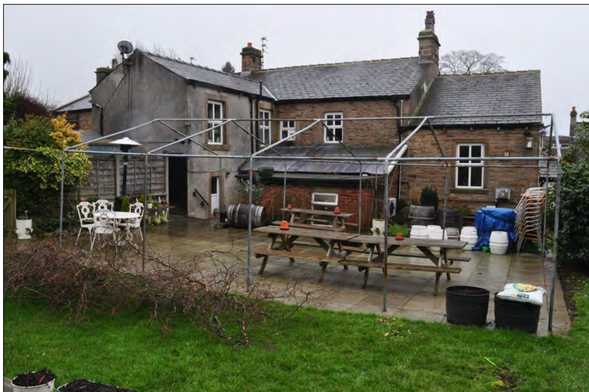
Photo 3: Rear of the pub, with steel frame of existing temporary shelter
