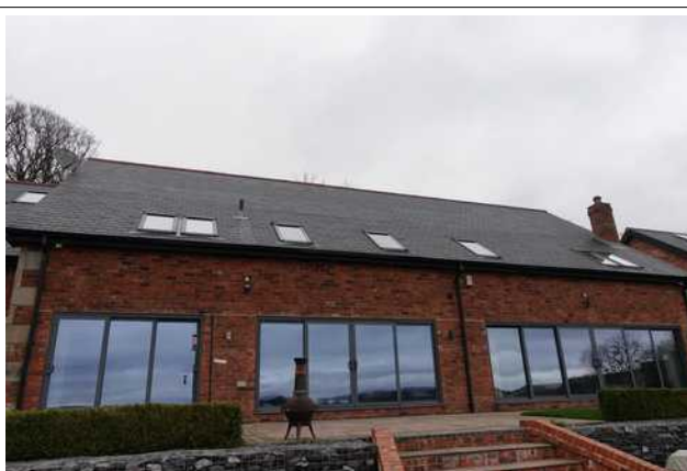
South facing facade
