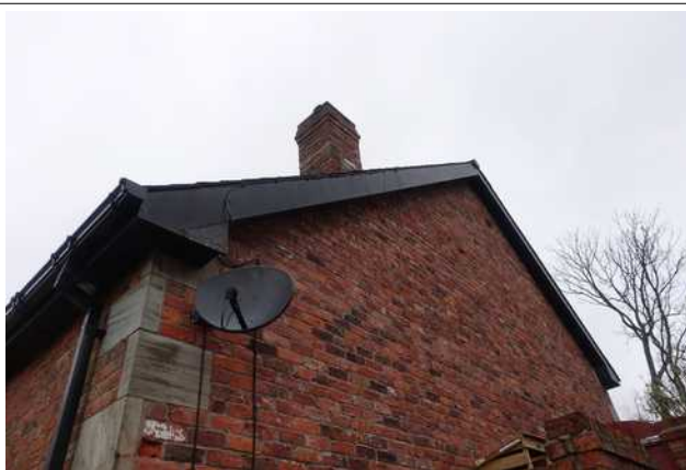
Eastern gable end
