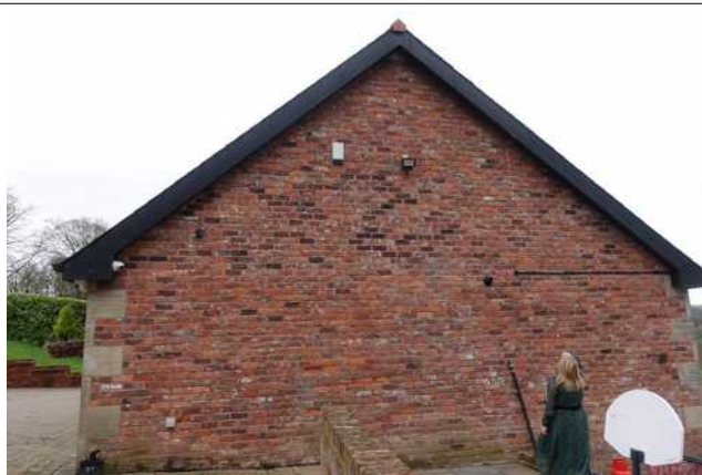
Western gable end
