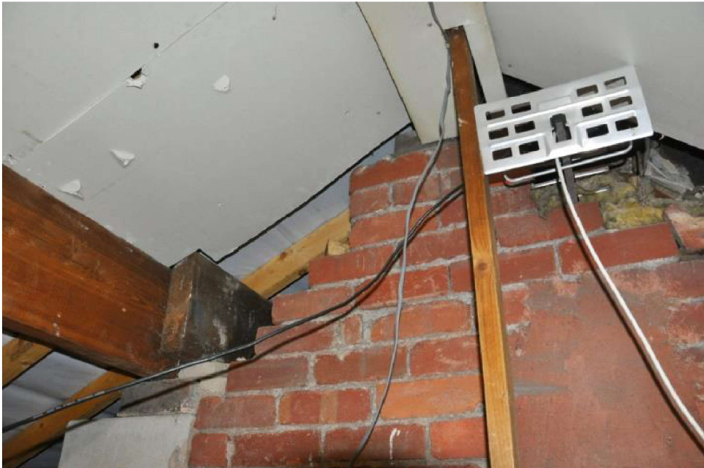
Image showing roof void with dividing brick wall, plaster boards and modern roof membrane roof liner
