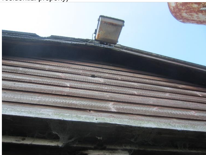
Photo 13: Timber planks at elevations of Building 1 (and 2)
