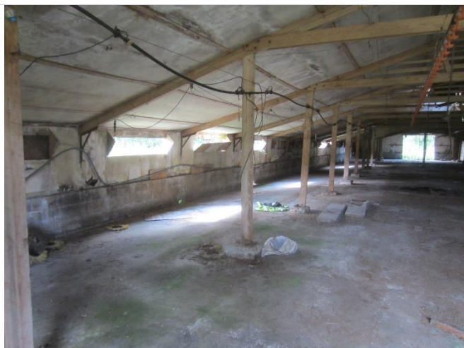
Photo 14: Interior of Building 1 showing well-pointed concrete block section of walls
