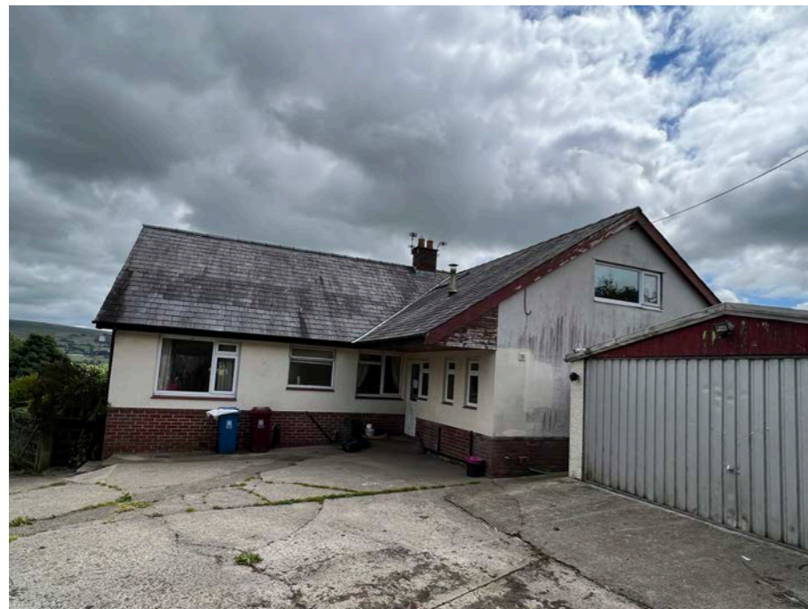
existing property - rear elevations
