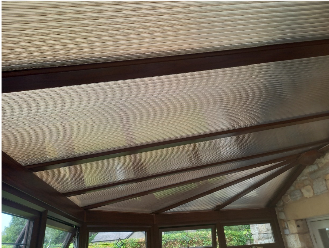
Conservatory with polycarbonate roof sheets with no gaps or voids for bats
