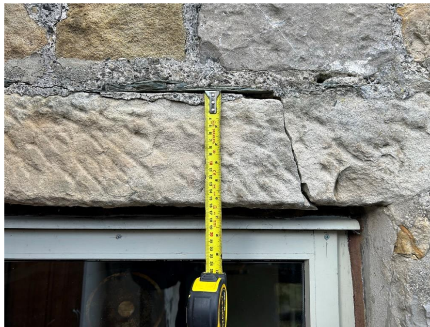
Photo 7: Broken window head
