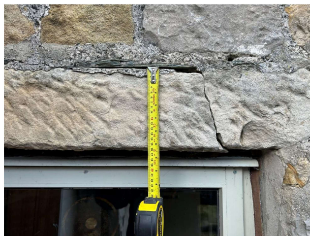
Photo 7: Broken window head
