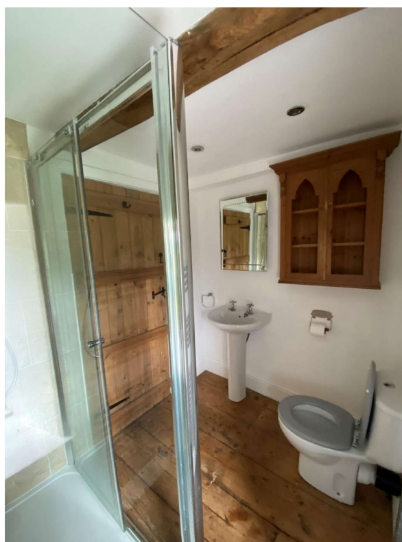
Photo 6: View across shower room proposed for retention, including wide floor boards and new plank door
