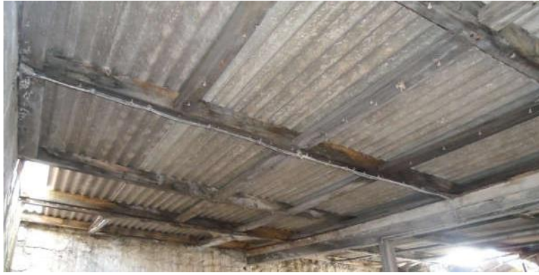
Photograph (2)- dilapidated roof structure of the lean -to.
