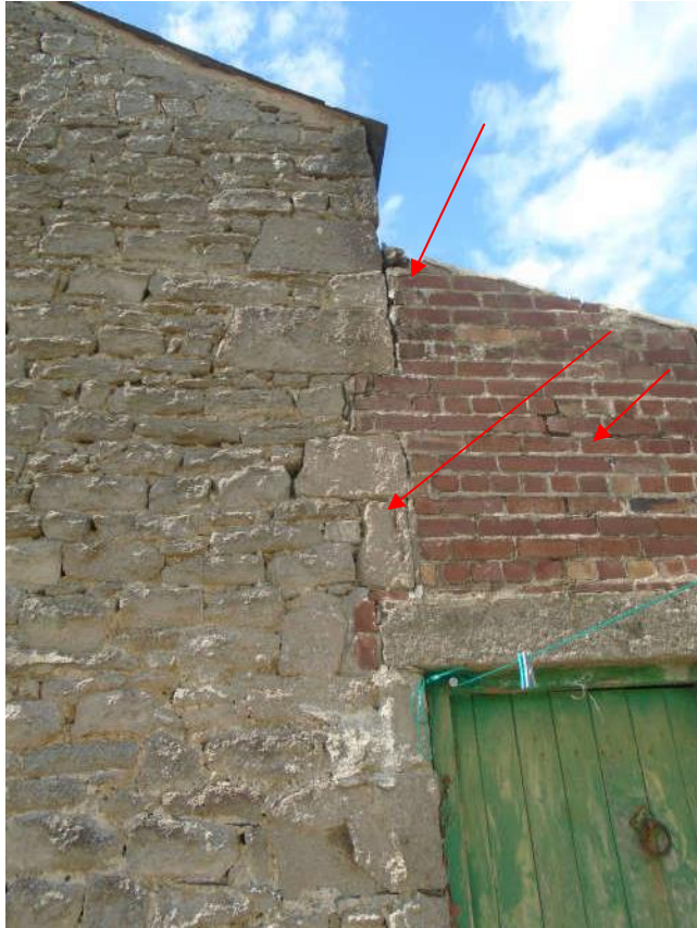
Photo (3) – East elevation cracks at lean -to abutment
