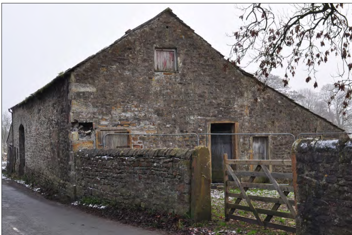
Photo 2: West end of barn, with doorways to stable, and shippon outshut (right)
