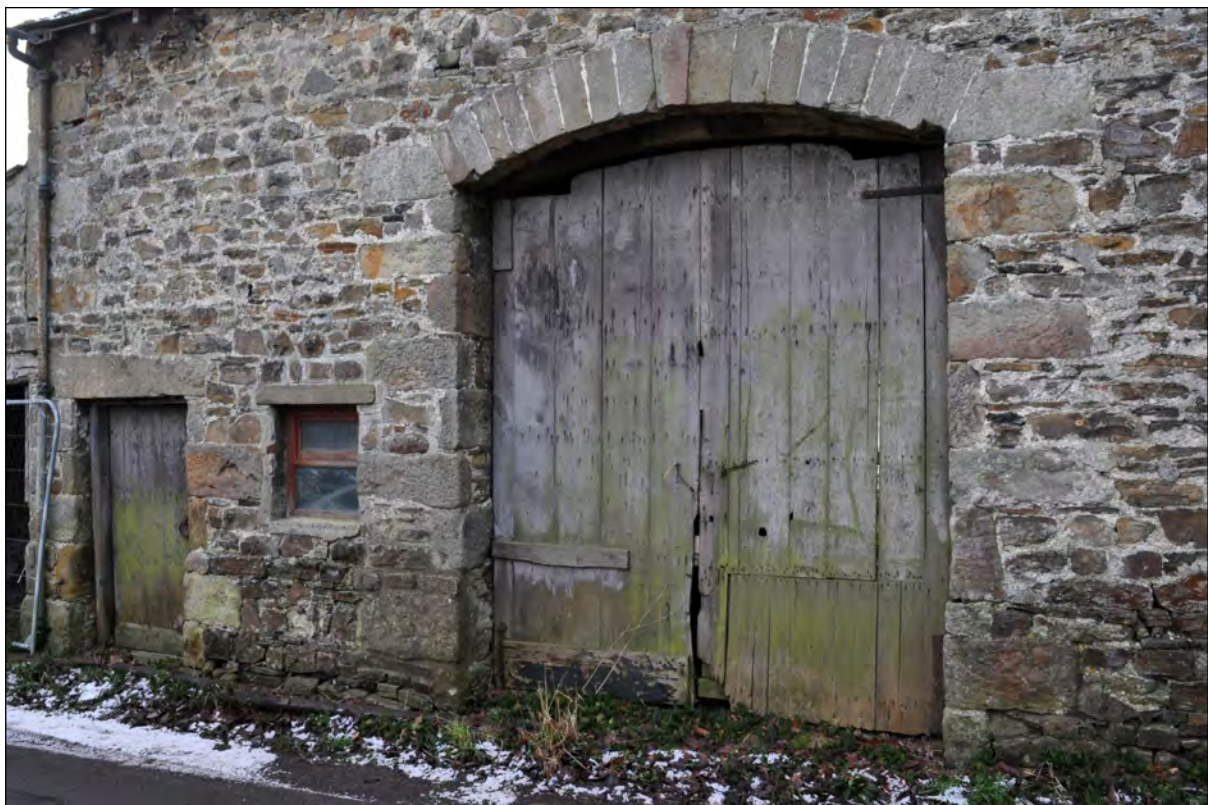
Photo 3: Detail of doorways and modern window opening in north side
