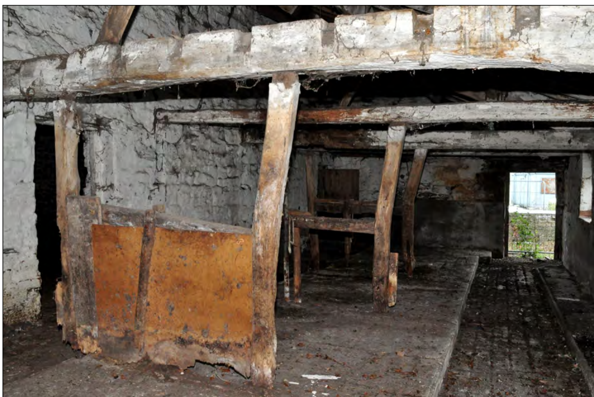
Photo 10: Interior of outshut shippon, looking east
