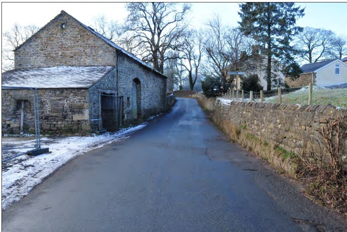
Photo 1: The barn, viewed along Grindleton Road. Lane Side farmhouse to right.
