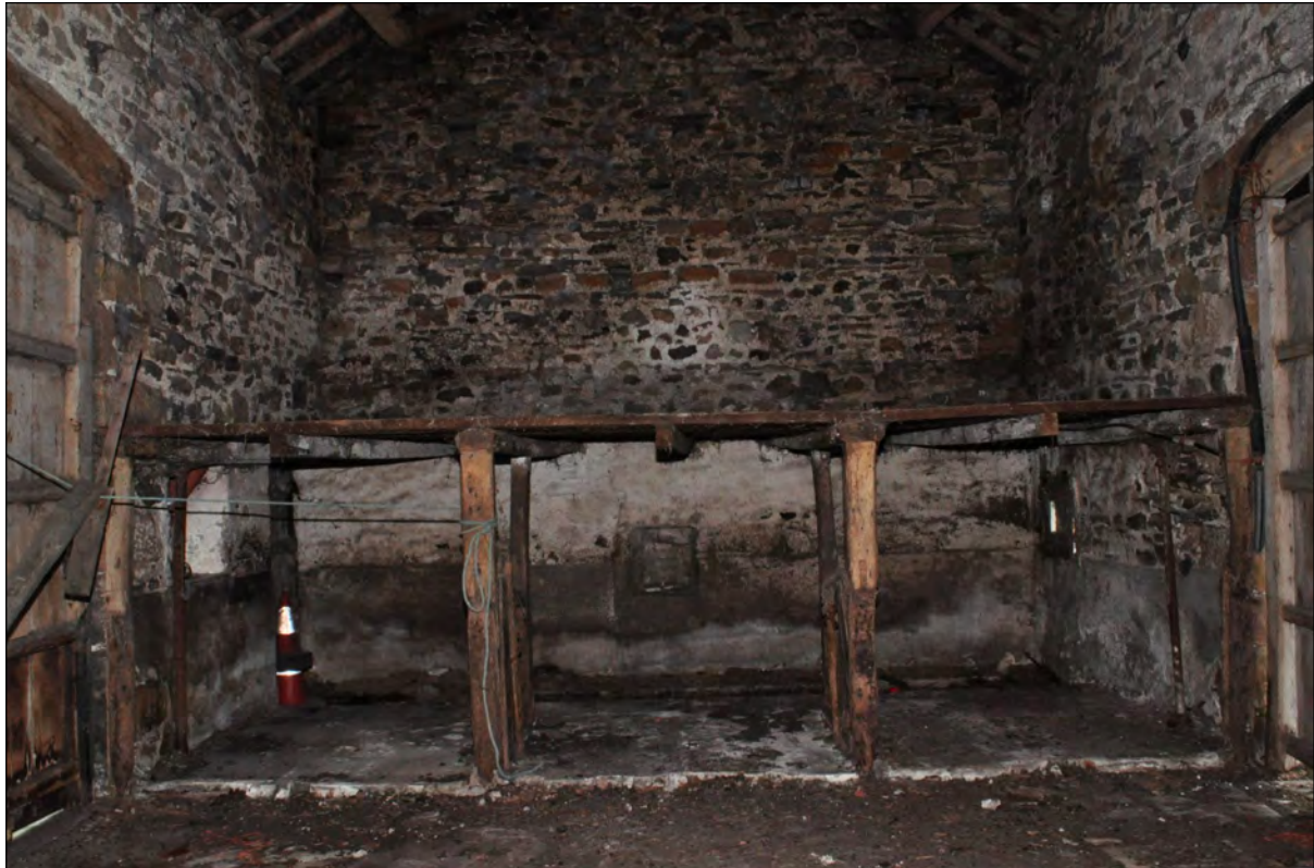
Photo 6: Shippon to east of threshing bay, with remains of timber structure
