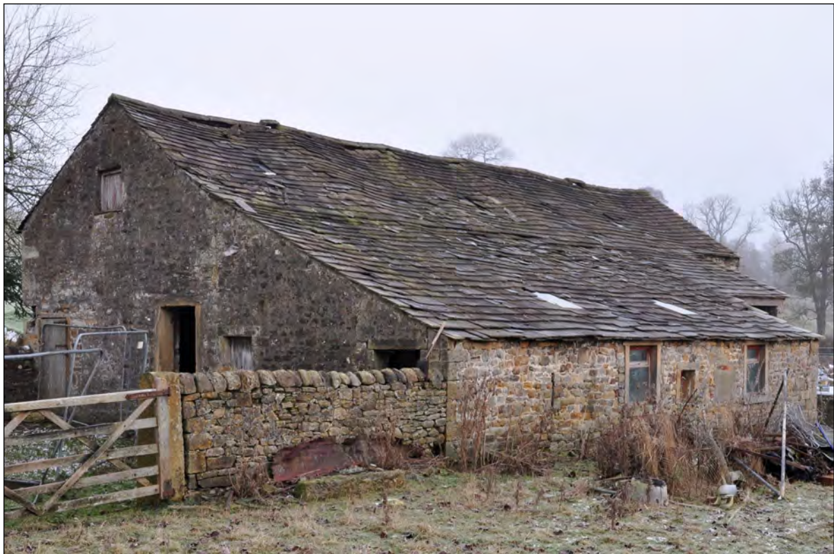
Photo 5: View from south-west, showing later shippon
