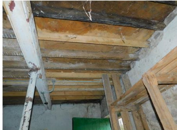
PHOTO 18 Underside of Central First Floor
