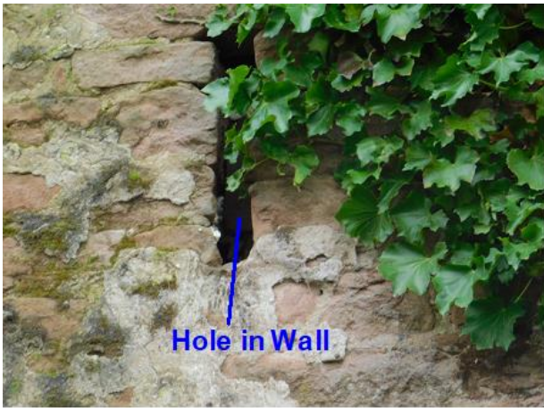
PHOTO 13 Part Northern Elevation
