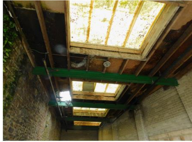
PHOTO 20 Underside of Extension Roof
