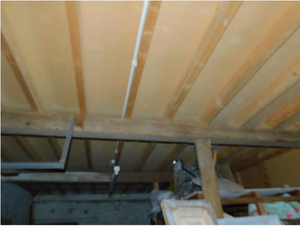
PHOTO 19 Underside of Southern First Floor
