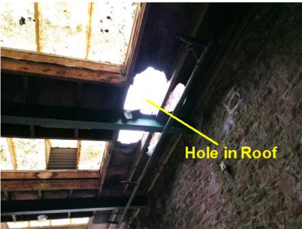
PHOTO 21 Underside of Central Extension Roof
