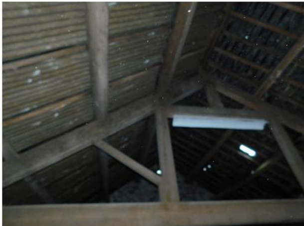
PHOTO 17 Underside of Central Roof
