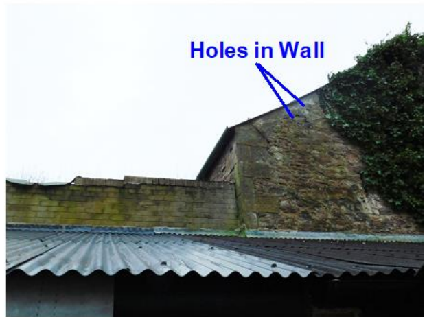
PHOTO 12 Upper North-western Corner
