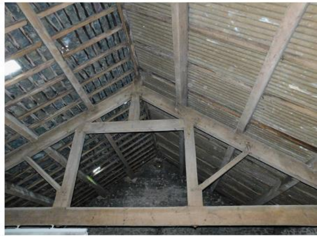
PHOTO 16 Underside of Northern Roof
