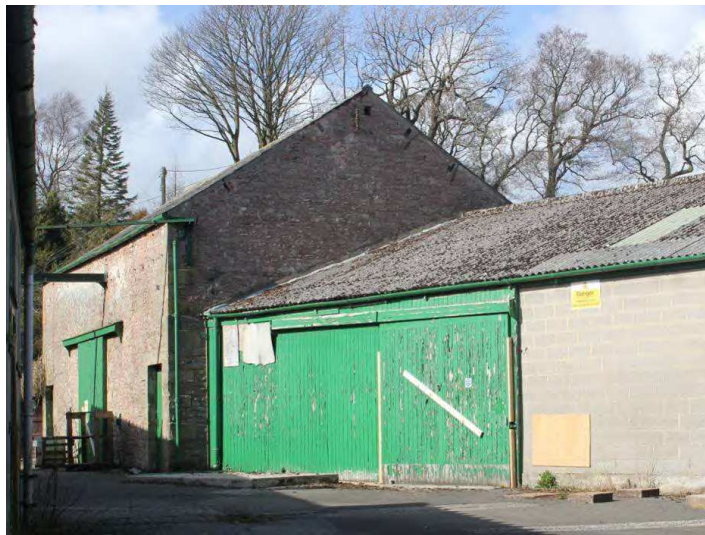
Fig 10—The Old Barn—OA North image (2015)
