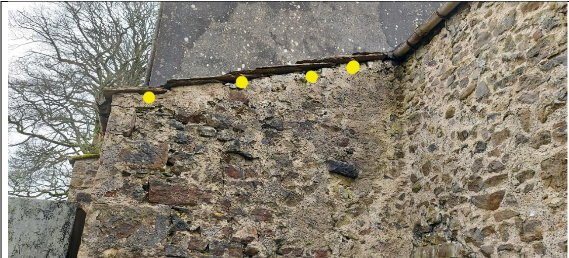
Building B2a – west elevation – missing mortar from edge tiles.
