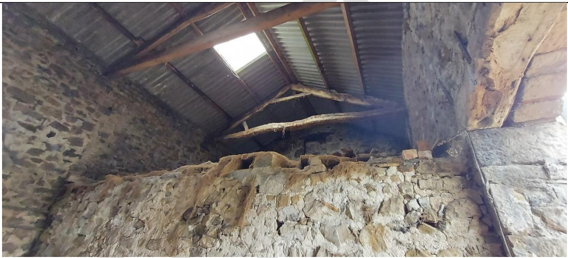
Building B2b – hayloft interior, potential for cavity bats.
