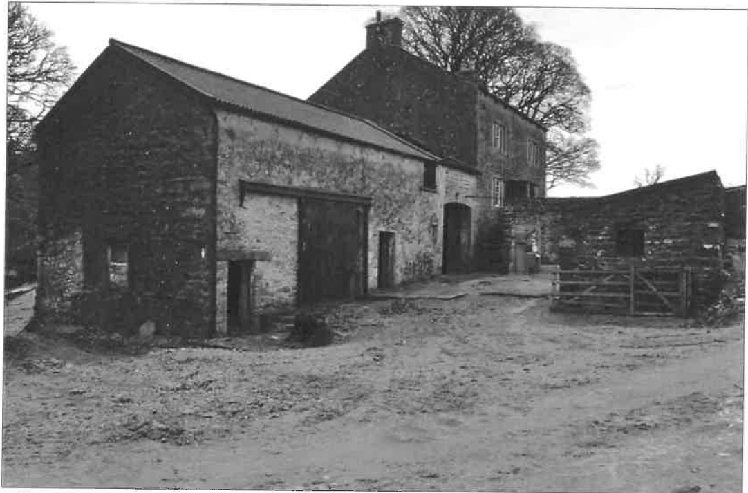
Photo 3: View of buildings from the south-west
