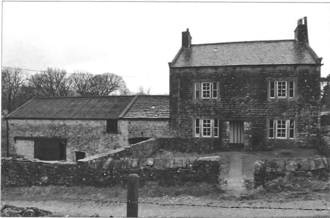
Photo 1: Front of farmhouse and adjoining buildings
