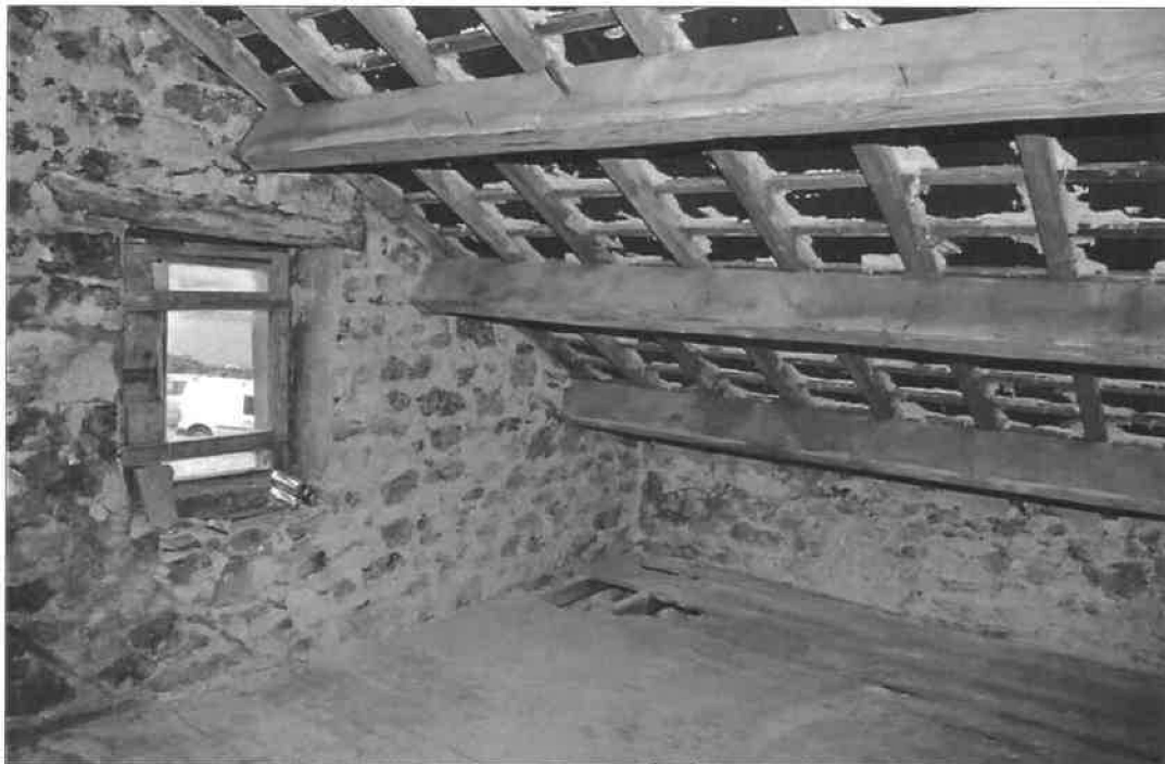
Photo 14: Attic, in south-east corner
