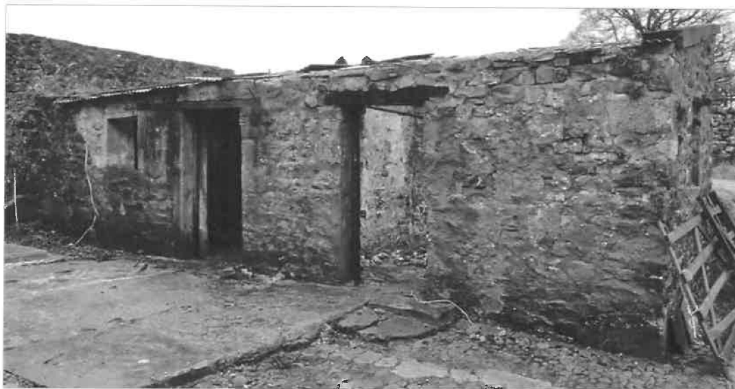
Photo 6: Outbuildings on south side of yard
