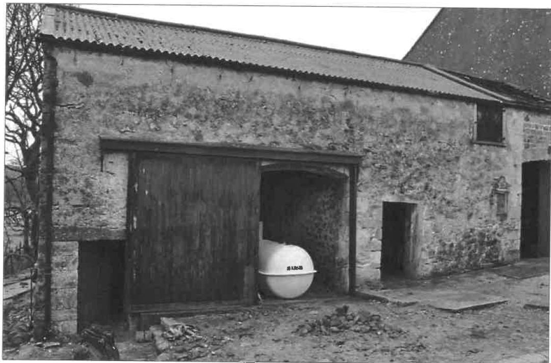
Photo 4: Front of barn
