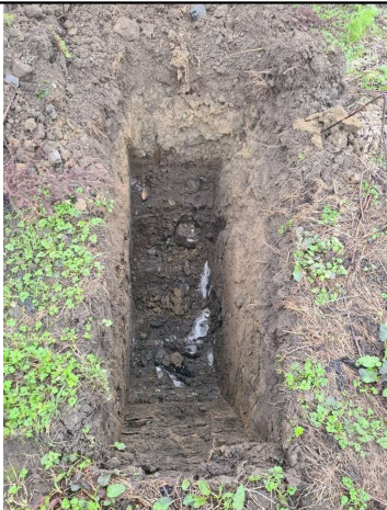
Soakaway 102/ Trial Pit 102
