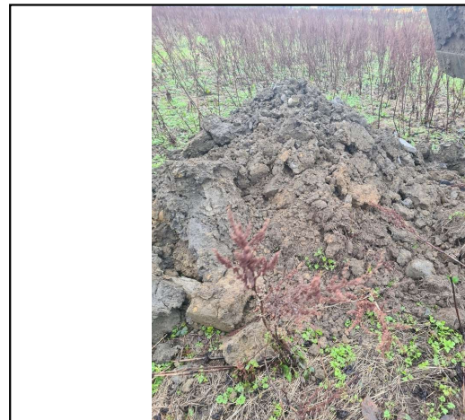
Soakaway 103/ Trial Pit 103 Spoil
