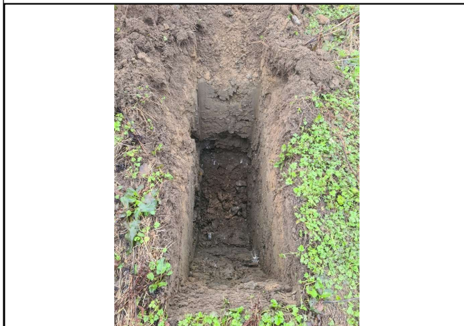
Trial Pit 103/ Soakaway 103
