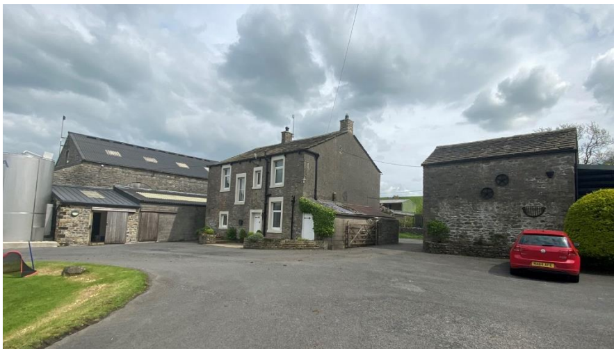
Photo 1: Barn (left), farmhouse (centre) and mistal (right)
