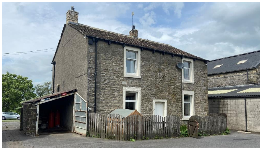
Photo 3: Rear south-east elevation of farmhouse
