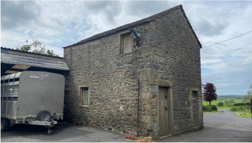
Photo 5: South-east elevation of mistal
