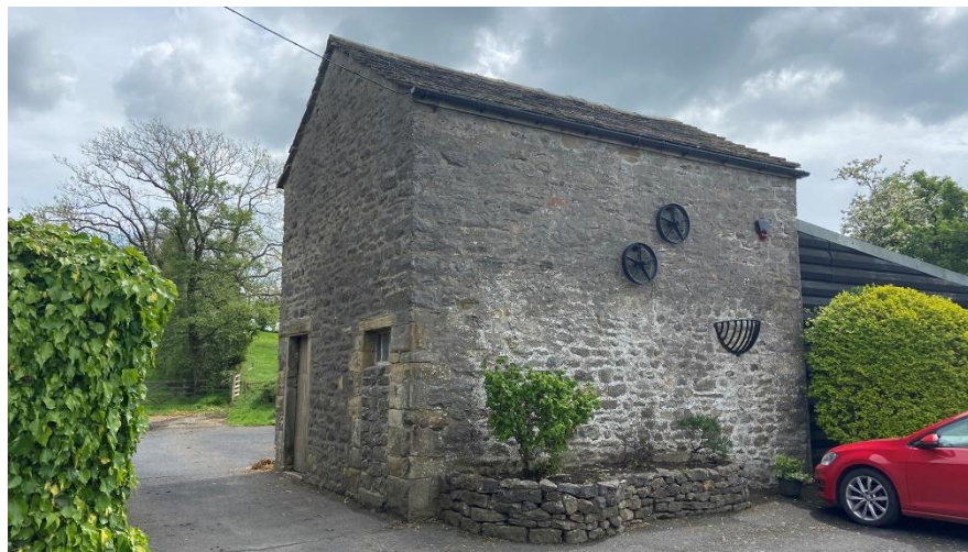
Photo 4: North-west elevation of mistal
