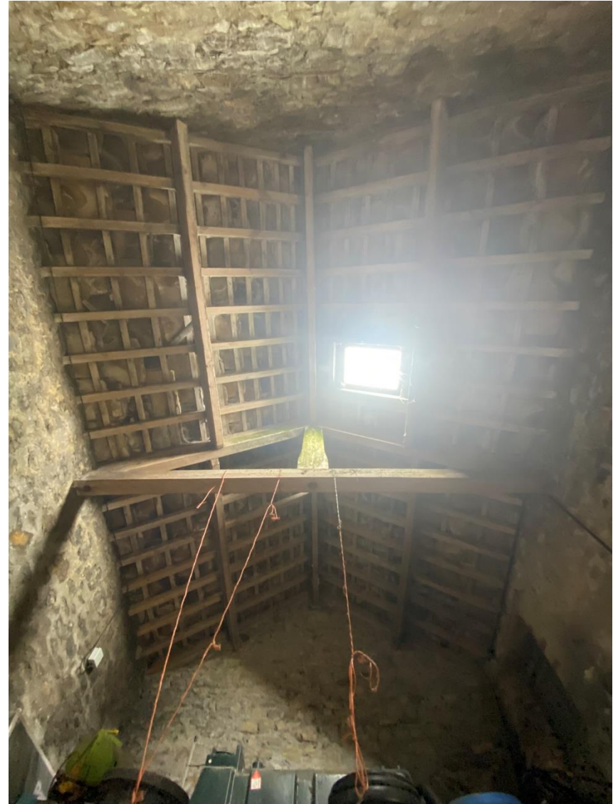
Photo 5: Mistal roof structure
