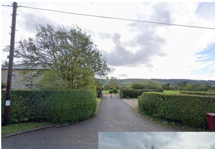
existing site entrance from highway
