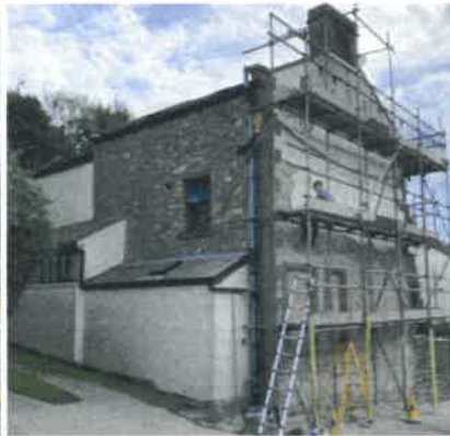
Rear ( north ) and side ( west ) elevation
