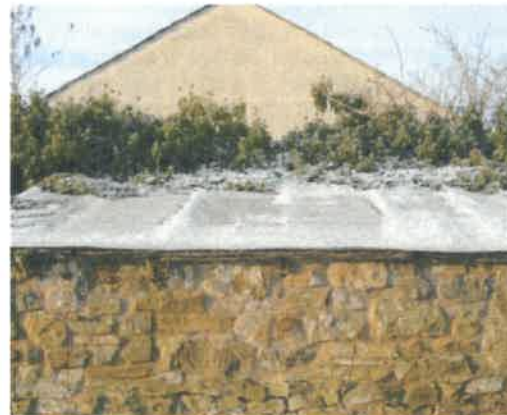
Outbuilding walls and house gable
