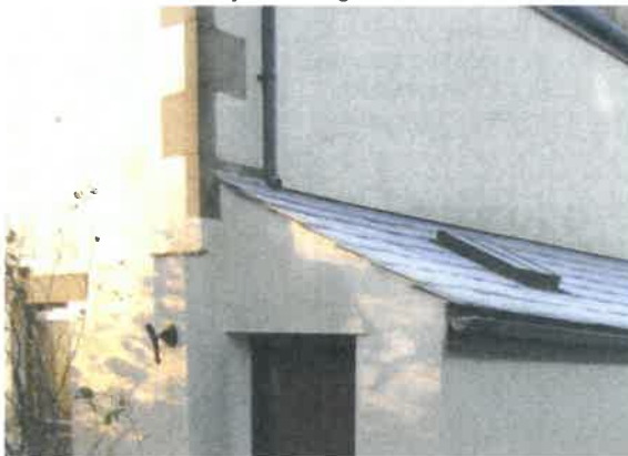
House gable and lean to walls
