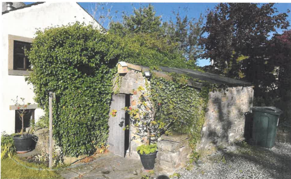
PL04 - Photograph of the existing south elevation of the outbuilding
