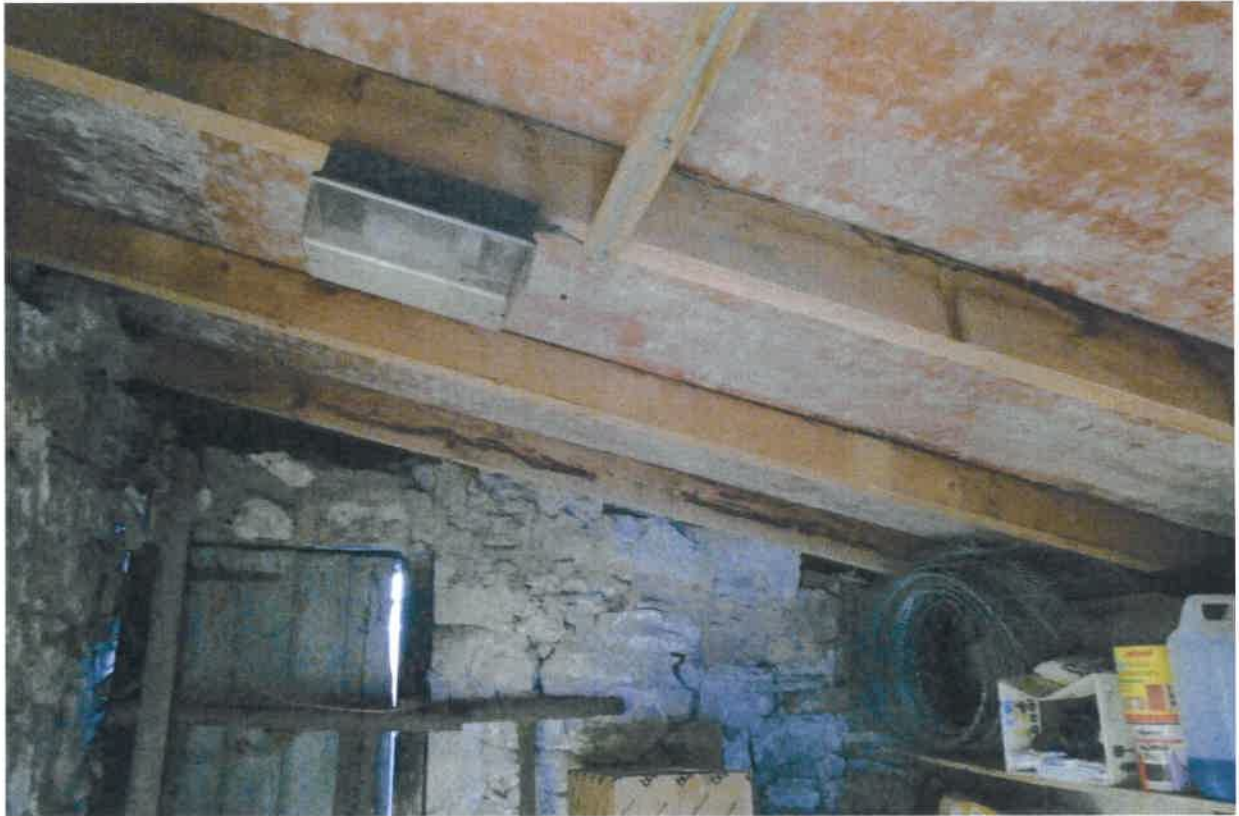
PL06 - Photograph inside the outbuilding, showing the modern roof structure.
