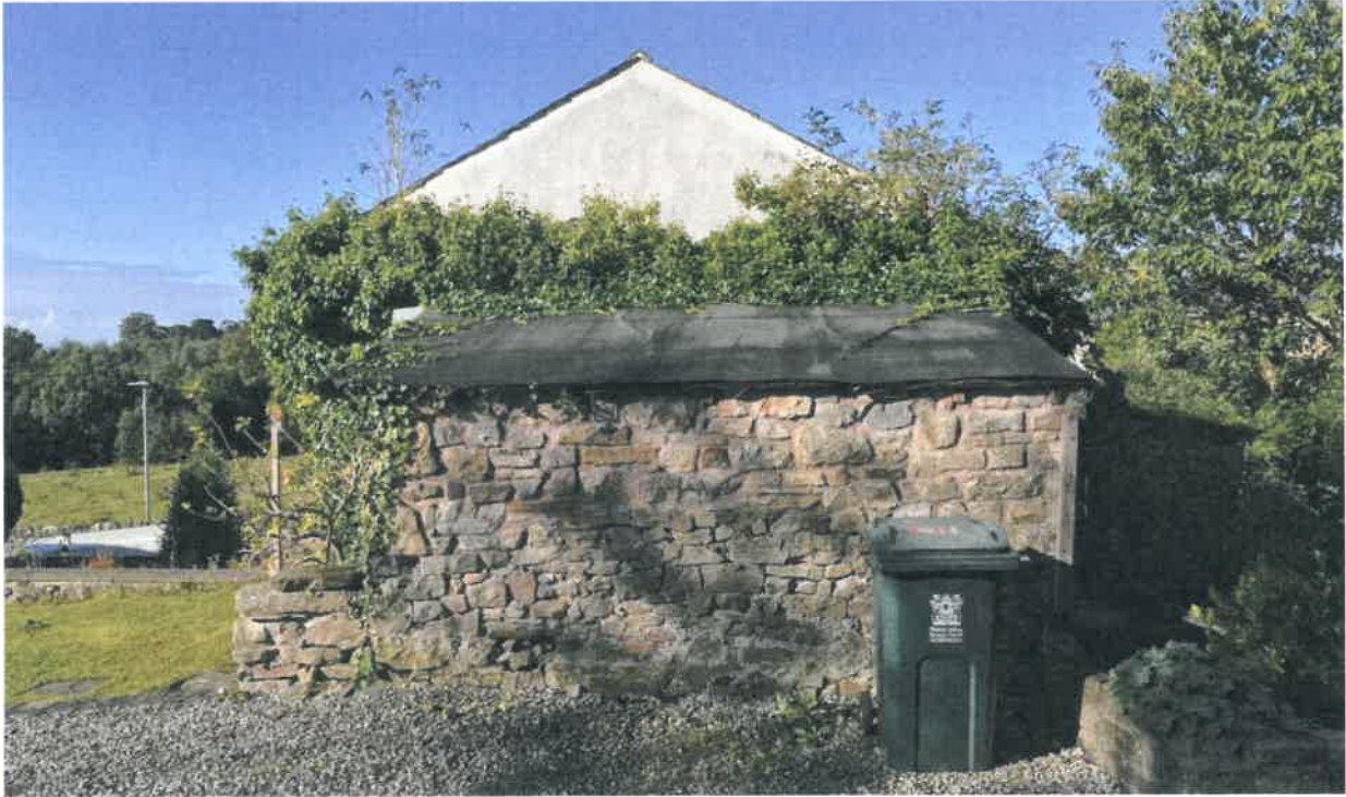
PL02 - Photograph of the existing east elevation of the outbuilding
