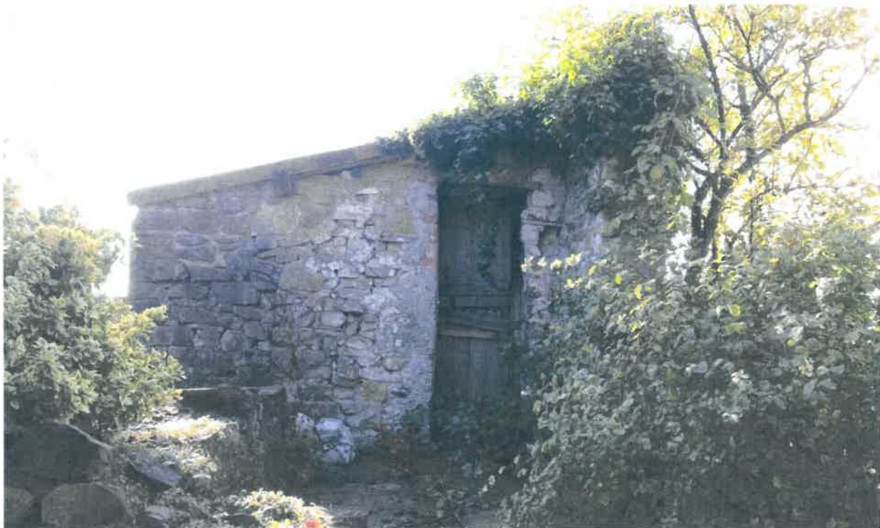
PL03 - Photograph of the existing north elevation of the outbuilding
