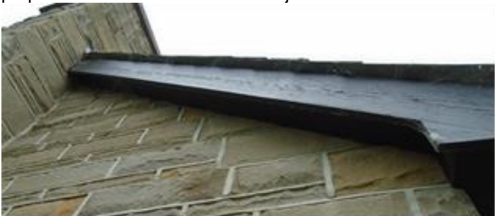
The extension gable barge board and soffit and slate abutment all in excellent condition and very tight fitting.
