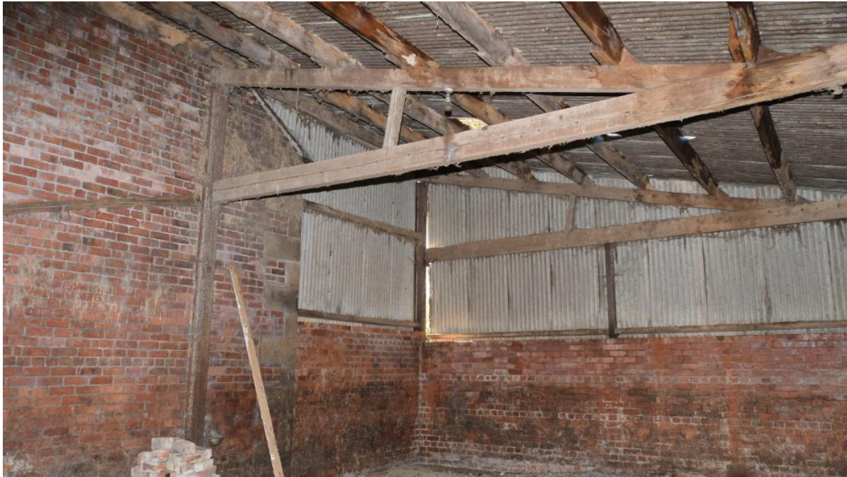
Internal view of hay barn
