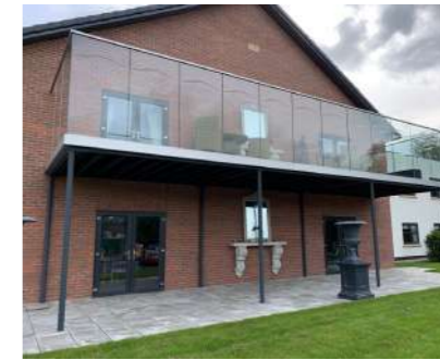
7. 1.8 metre High Glass Balustrade
