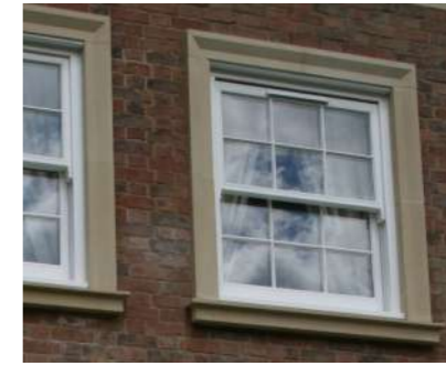
3. Reconstituted Stonework Window Surrounds
