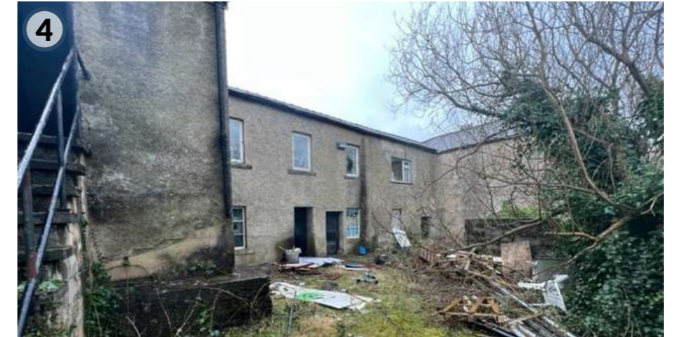
Image 4 - 2 storey building providing access to courtyard on north boundary.
