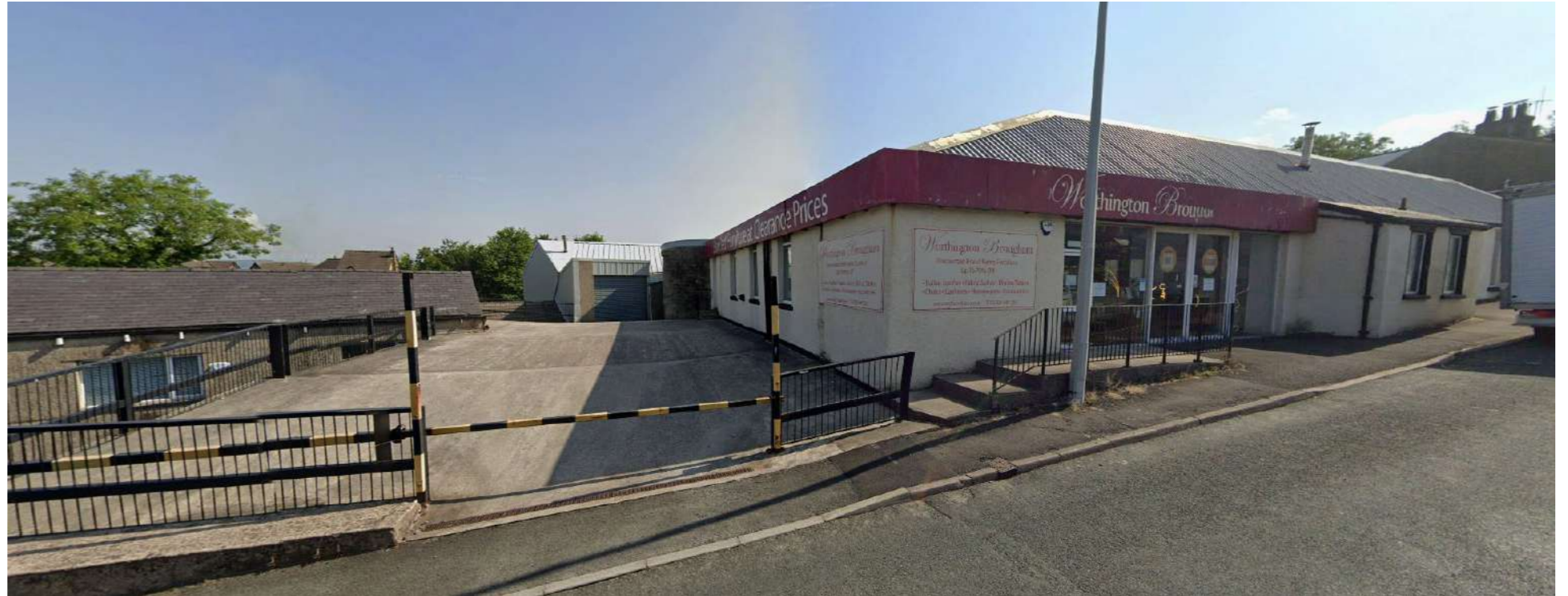
Approach Three - South west boundary showing existing building and loading bay area.
