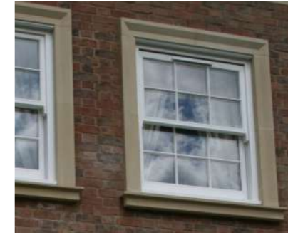
3. Stonework Window Surrounds
