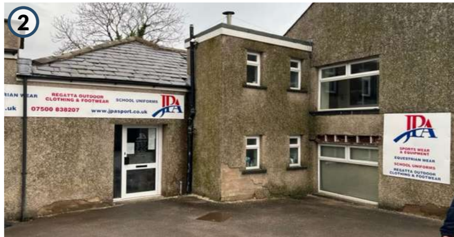
Image 2 - Building situated off loading area (1 to 2 storey unit).
