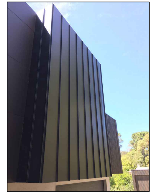
Proposed Example of Standing Seam Cladding
