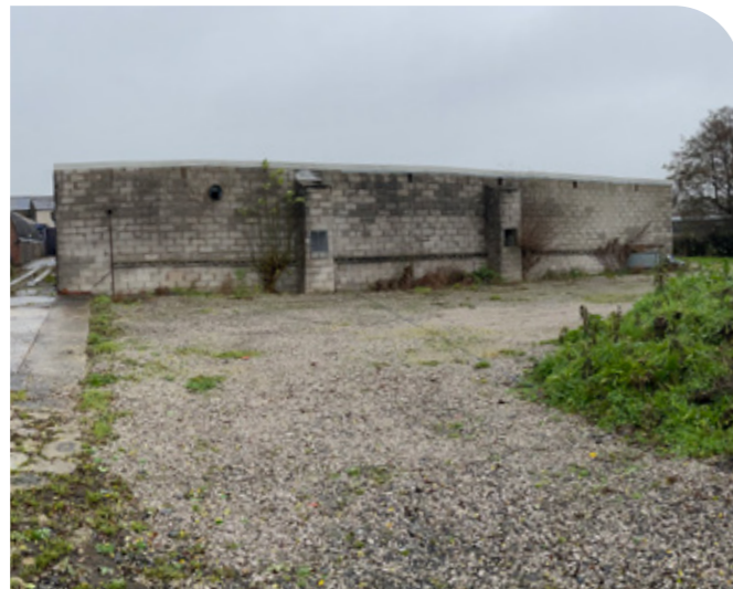
Figure 1.1: Existing south elevation
