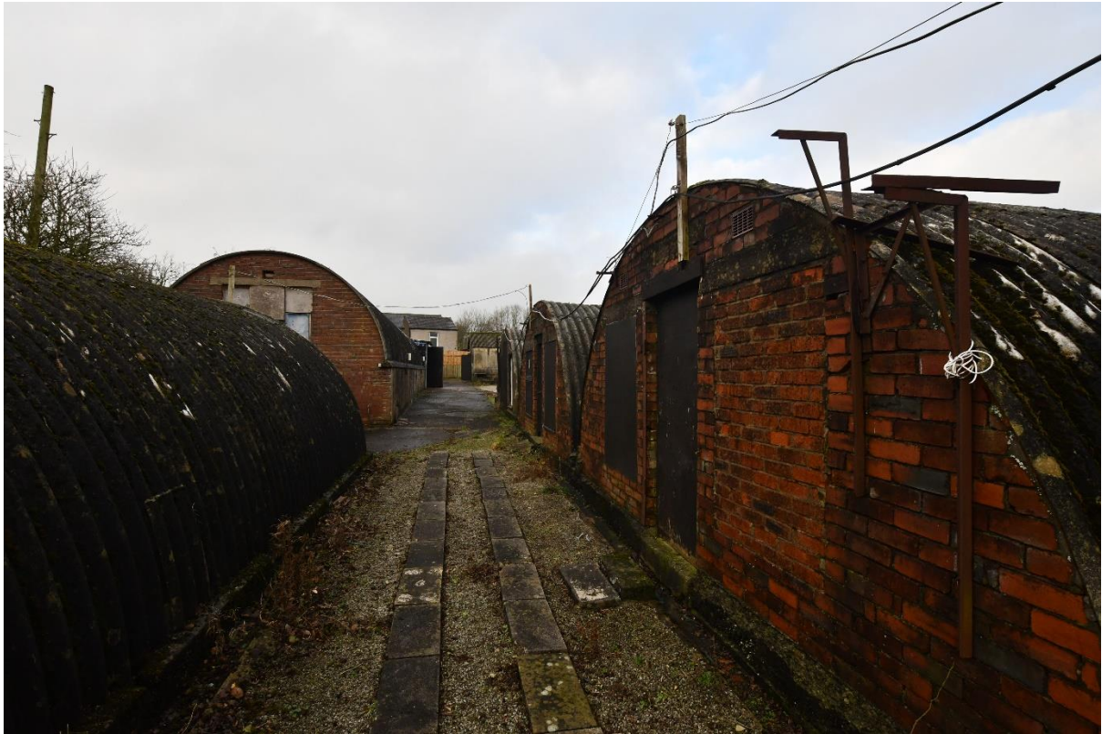
Image 5 Looking north through the various buildings
