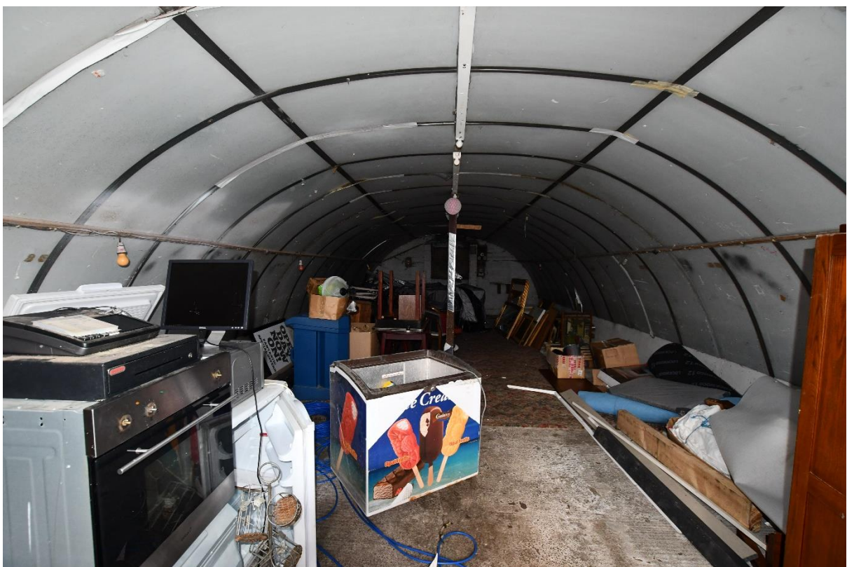
Image 4 Internal structure of large workshop target building
