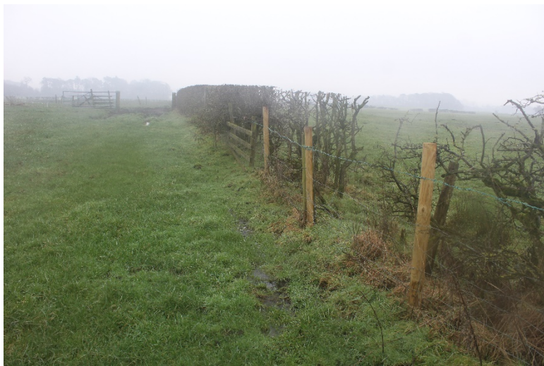
TN4 Defunct hedge of hawthorn to south-west, with fencing
