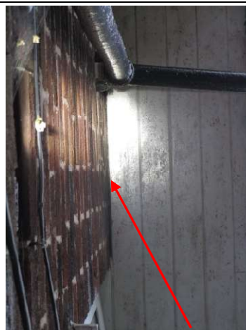
Photo 6: Building A – example of gap between soffit and wall.
