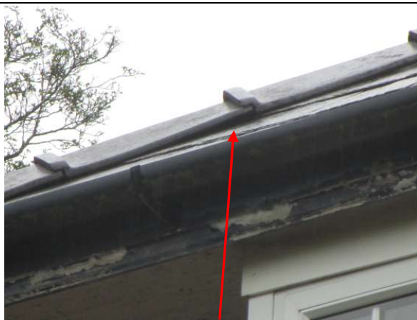
Photo 7: Building A – gap at ridge tile.
