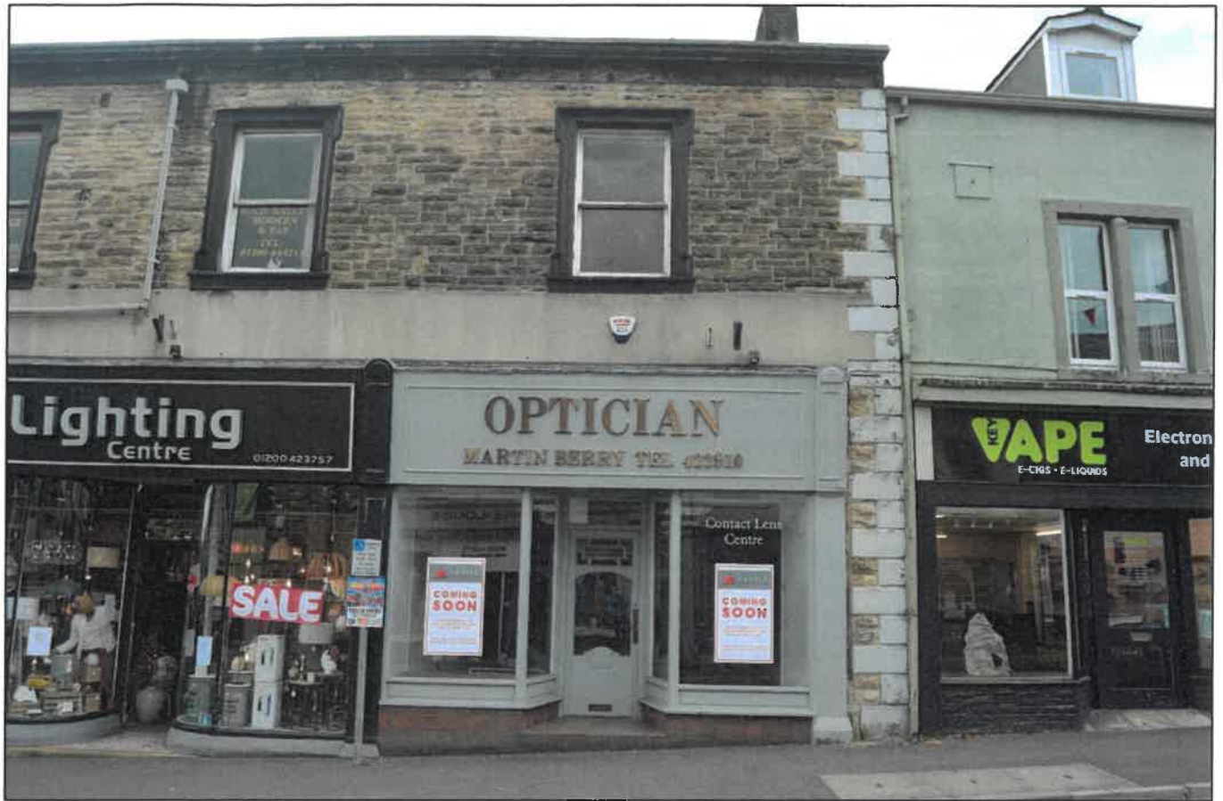
PL03: View of the front east facing elevation of 12 Moor Lane.
