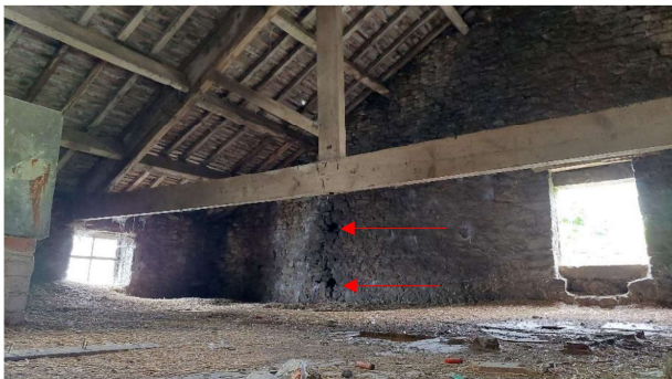
Photograph 12: Mezzanine in the eastern half of the building. Gaps in the stonework potentially provide suitable bat roosting opportunities.
