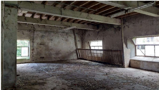
Photograph 10: Eastern room in the building. Presumed to have been used to house livestock.
