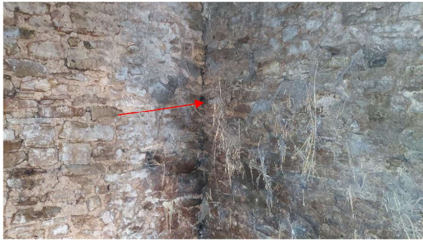
Photograph 14: Gaps in the south western corner were subject to endoscope but no bats recorded.
