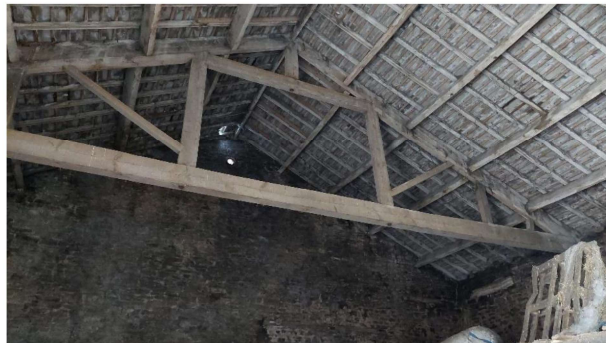
Photograph 8: Internal view of the roof frame and tiles.
