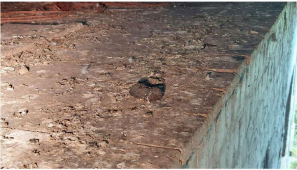
Photograph 17: Example of pellet recorded on the building's eastern mezzanine.
