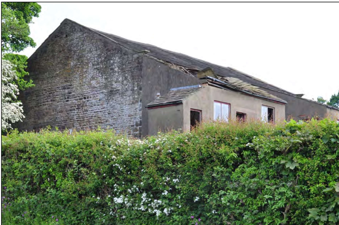
Photo 4: View of barn from Simonstone Lane, looking north-east
