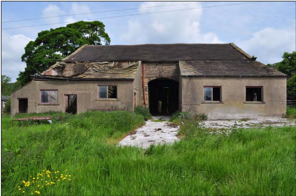
Photo 5: South side of barn, with mid twentieth century brick-built outshuts either side of arched cart entrance
