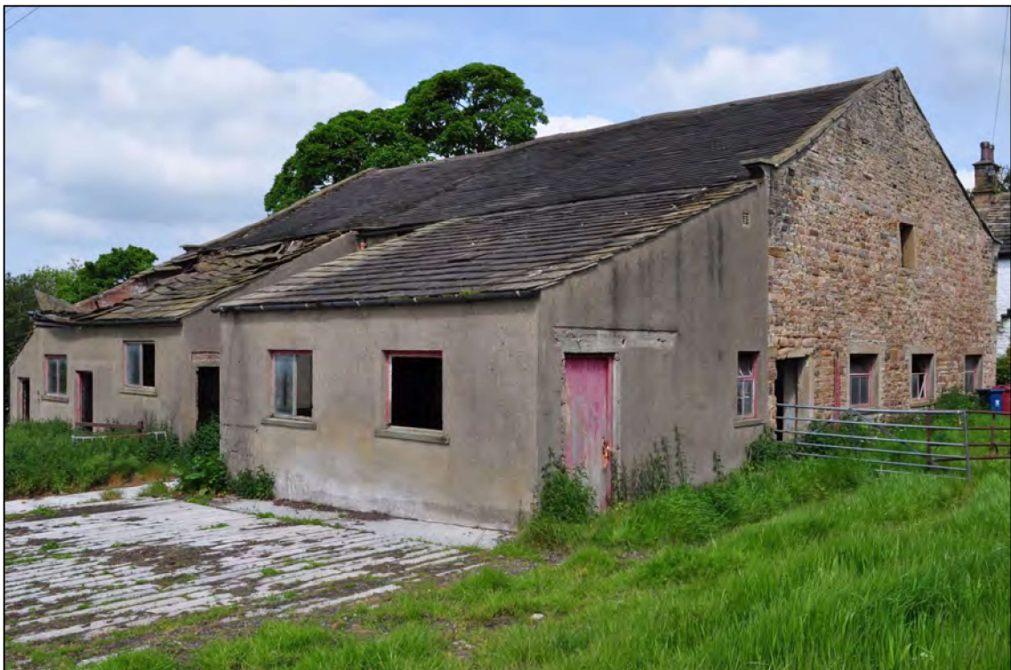
Photo 6: View of barn, looking north-west
