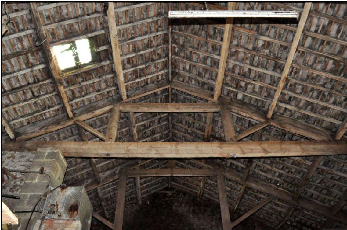
Photo 10: Roof trusses over barn
