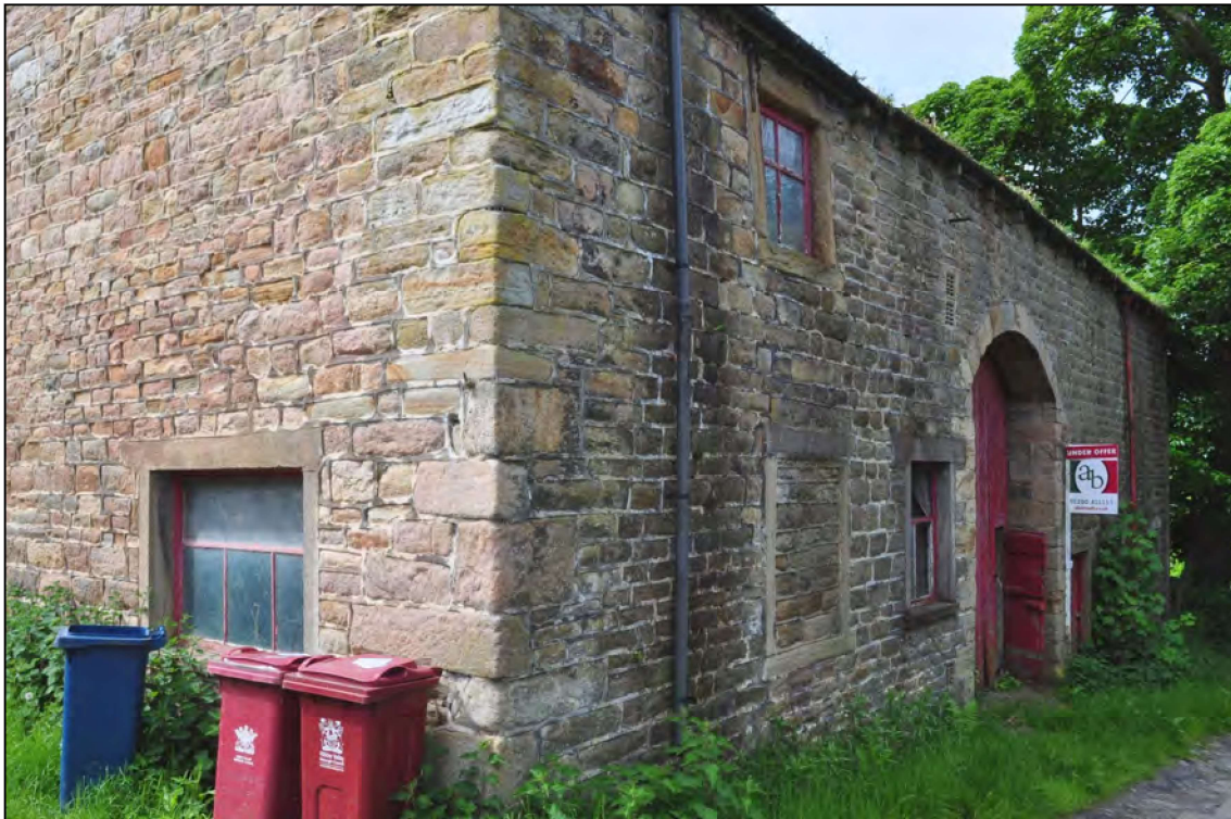
Photo 3: North elevation of barn
