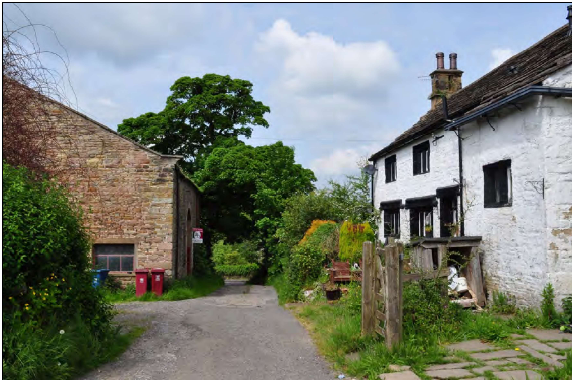
Photo 1: The barn (left) in relation to the listed building (right). Looking west, down towards Simonstone Lane
