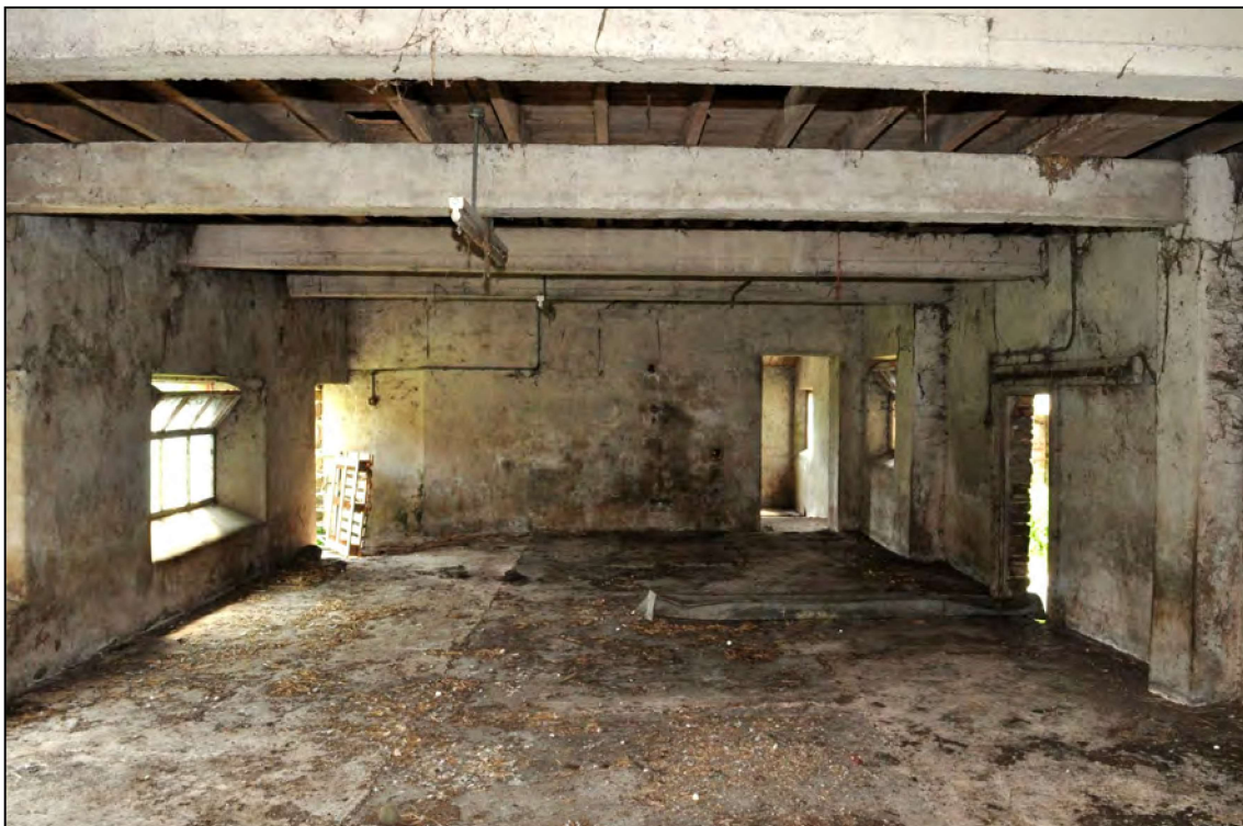
Photo 9: Modern shippon in east end of barn, with concrete beams over
