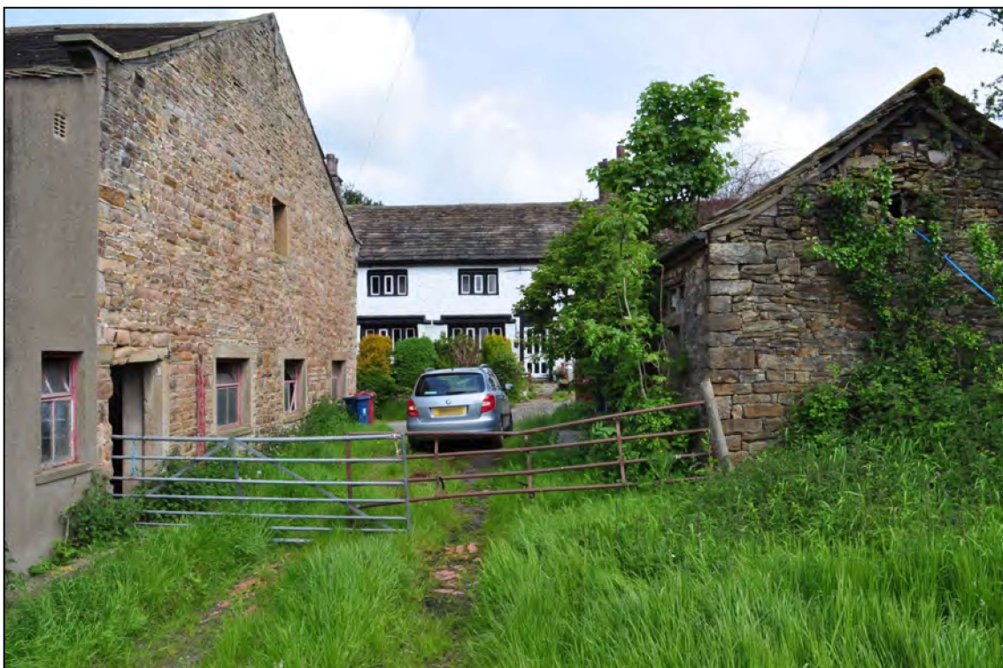
Photo 2: East gable of barn (left), outbuilding (right), and listed building (centre)
