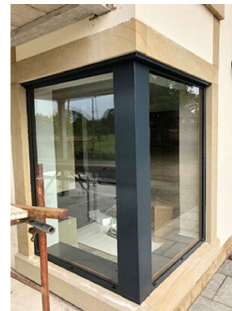
Powder coated aluminium window frames. Colour Anthracite Grey (RAL 7016)
