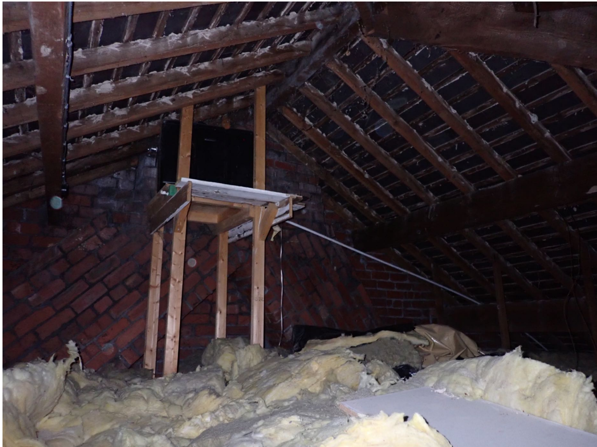
3.2a – The roof void.
