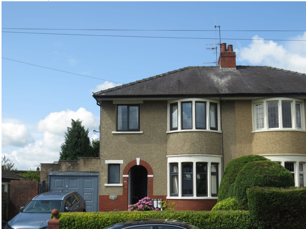
3.1a – The front of the house.
