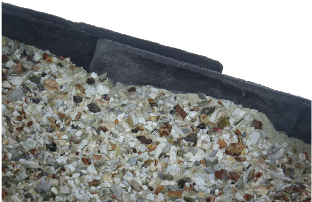
8 – End tiles at the verges are sealed with cement.
