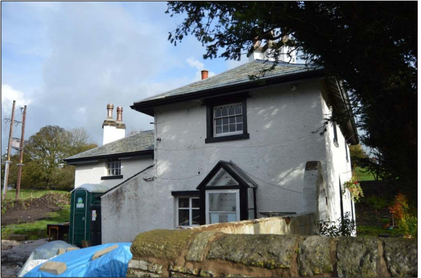
PL07: View of The Priory from the west.
